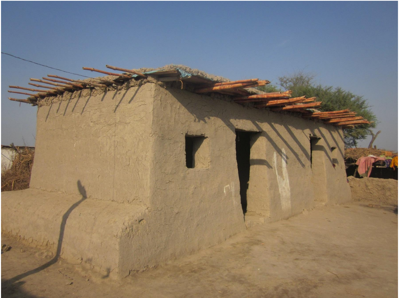
EMERGENCY SHELTER KIT reused in housing construction
