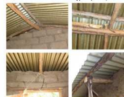
Added Tie-down of roof
