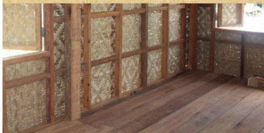
Sawali Wall clipped with 1"x2" lumber on the outside.
