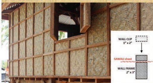
Sawali Wall clipped with 1"x2" lumber on the outside.
