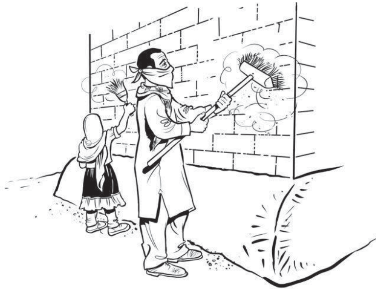
Fig 93: Brush walls to remove dust and debris
