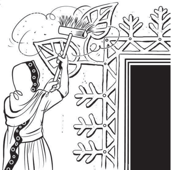
Fig 106: Brush down the walls to remove dust and debris, prior to wetting and applying lime wash
