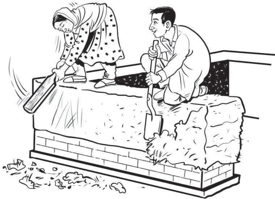
Fig 88: Cob wall making and shaping
