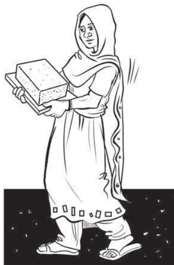
Fig 82: Careful handling and carrying of the newly made block (unless the block is demoulded in situ onto a flat, shaded surface)
