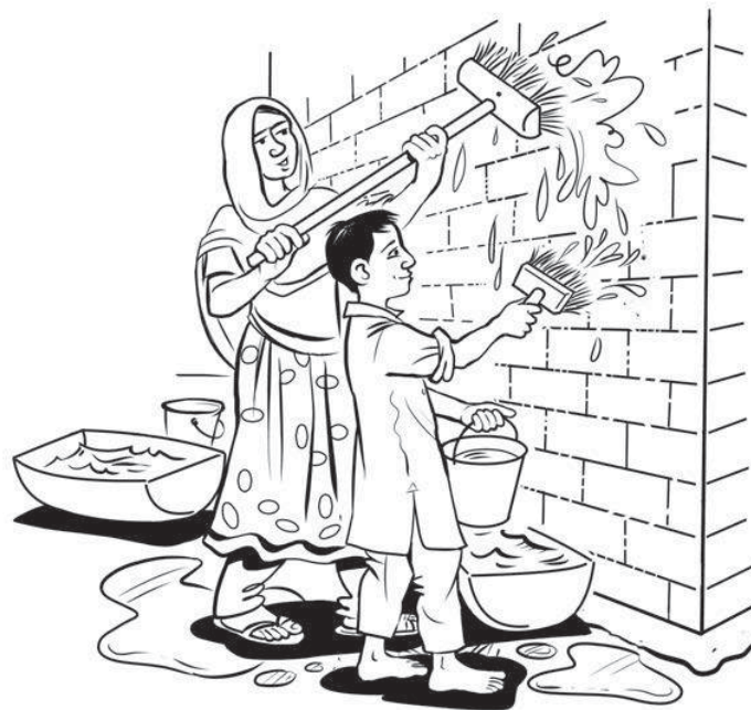
Fig 95- Wet the Walls before applying render
