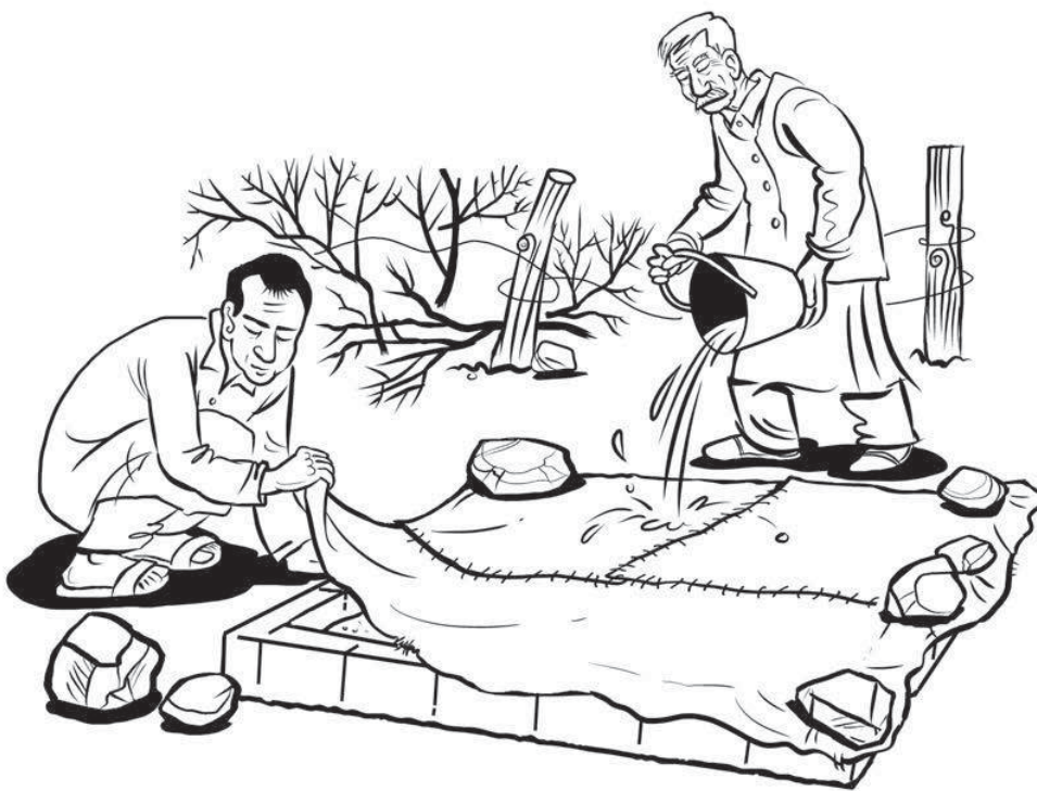
Fig 34: Keep the lime putty clean by keeping the putty settlement tank covered
