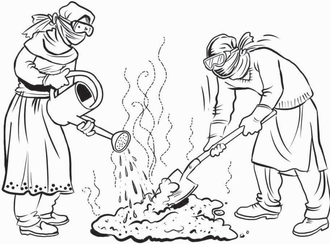
Fig 57: Hot Mixing - add minimum water
