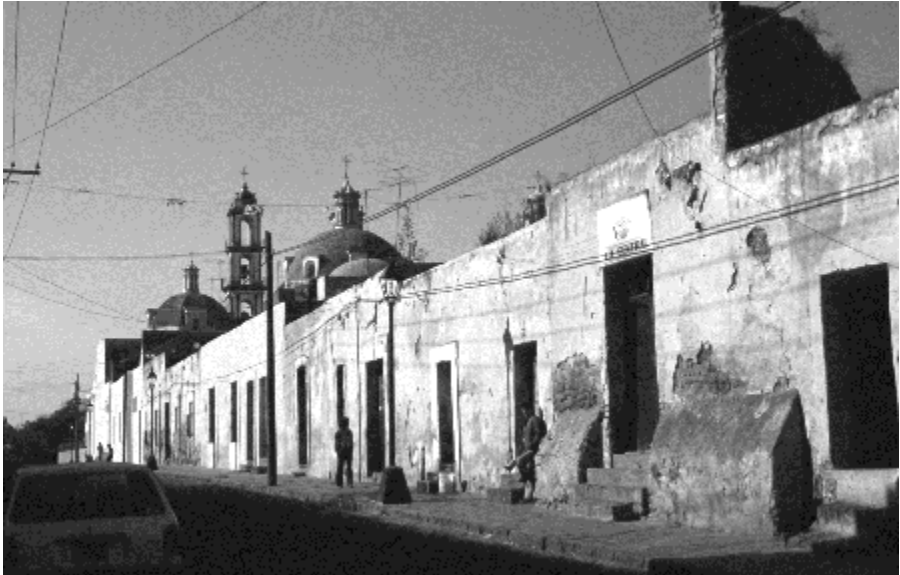
Photograph 7: Deteriorating rental housing in inner-city Puebla, Mexico
