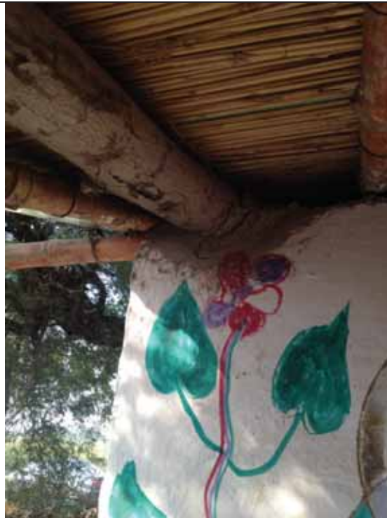
Photo 6 CESVI, Choudri Majeed Gihuman, Mirpur Khas Large timber beams span on to walls with no way of spreading the load
