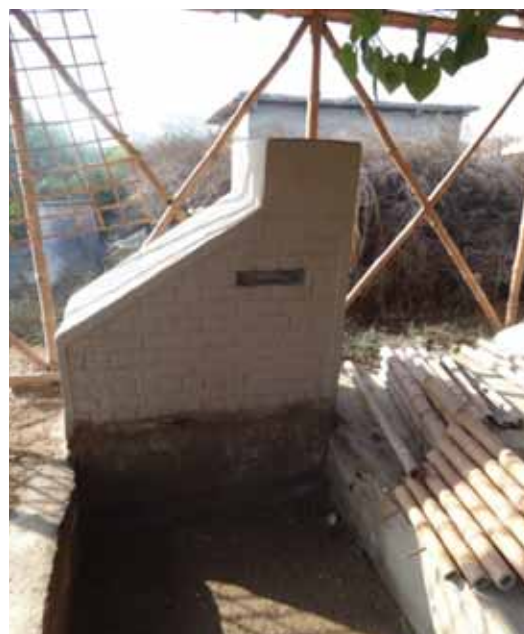
Photo 10 Heritage Foundation, Tando Allah Yar Full scale section through an adobe brick foundation for training purposes
