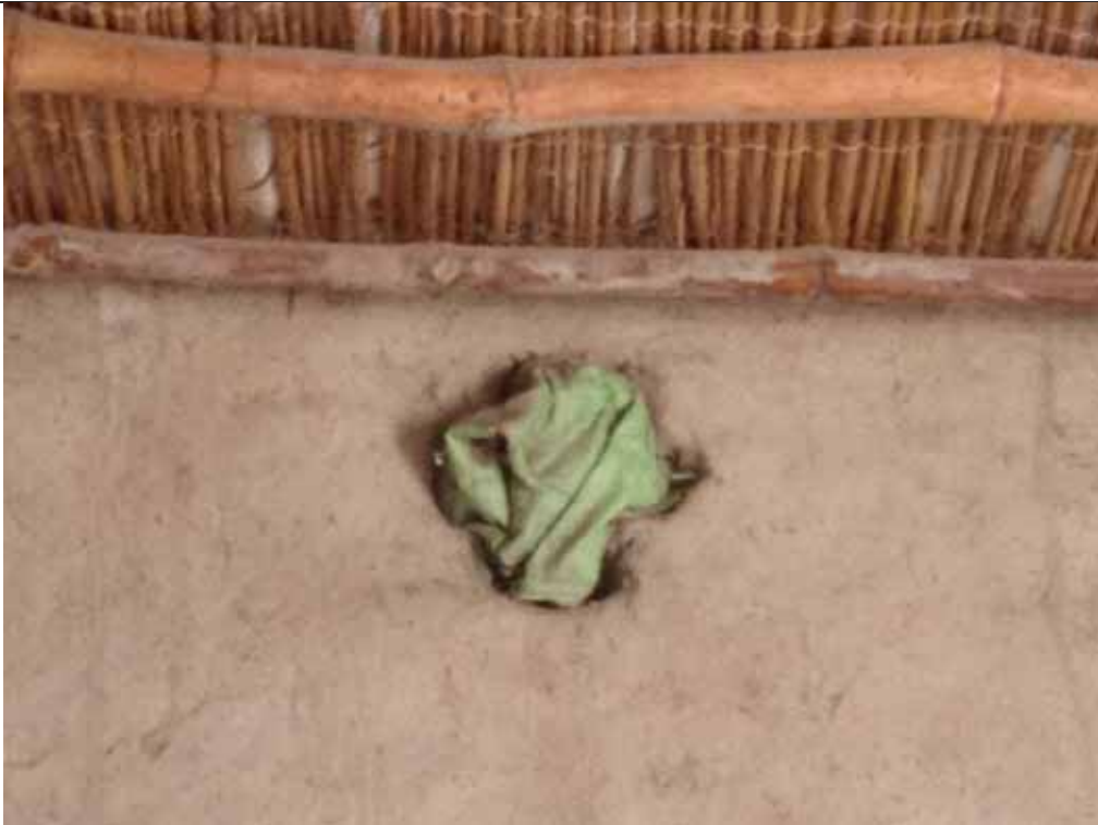
Photo 15 IOM, Jacobabad, Taulka Thulabab Ventilation holes covered up to stop birds nesting.
