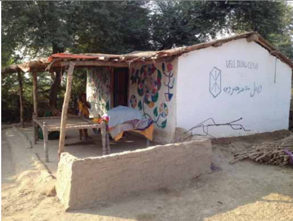
Photo 5 CESVI, Choudri Majeed Gihuman, Mirpur Khas Adobe Shelter Verandah extension using materials (bamboo/ timber) supplied by CESVI
