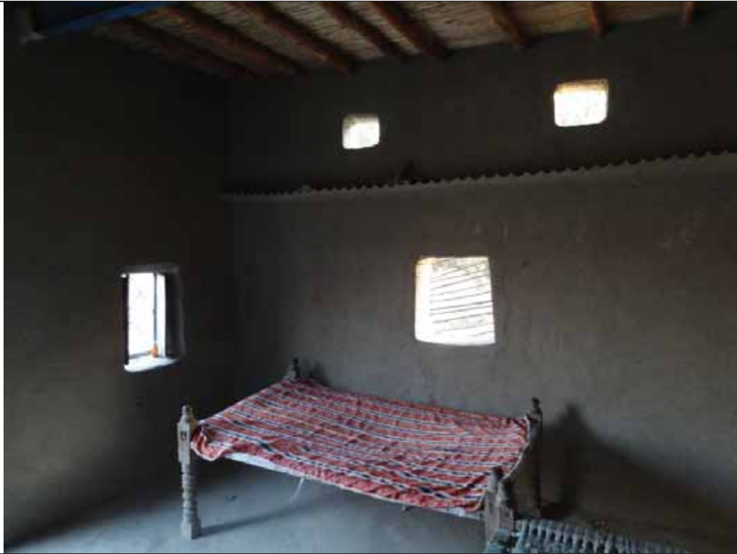
Photo 11 HANDS, Umerkot, Attar Mohammed Palli Good sized openings to allow for light and cross ventilation with thick mud walls which help maintain the internal temperature
