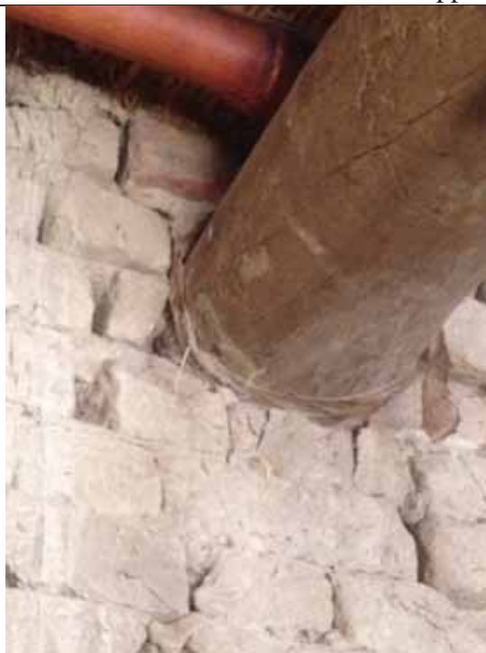
Photo 8 IOM, Shikarpur Large beams used for roof of extension connected to thin brick wall and crushing the brick
