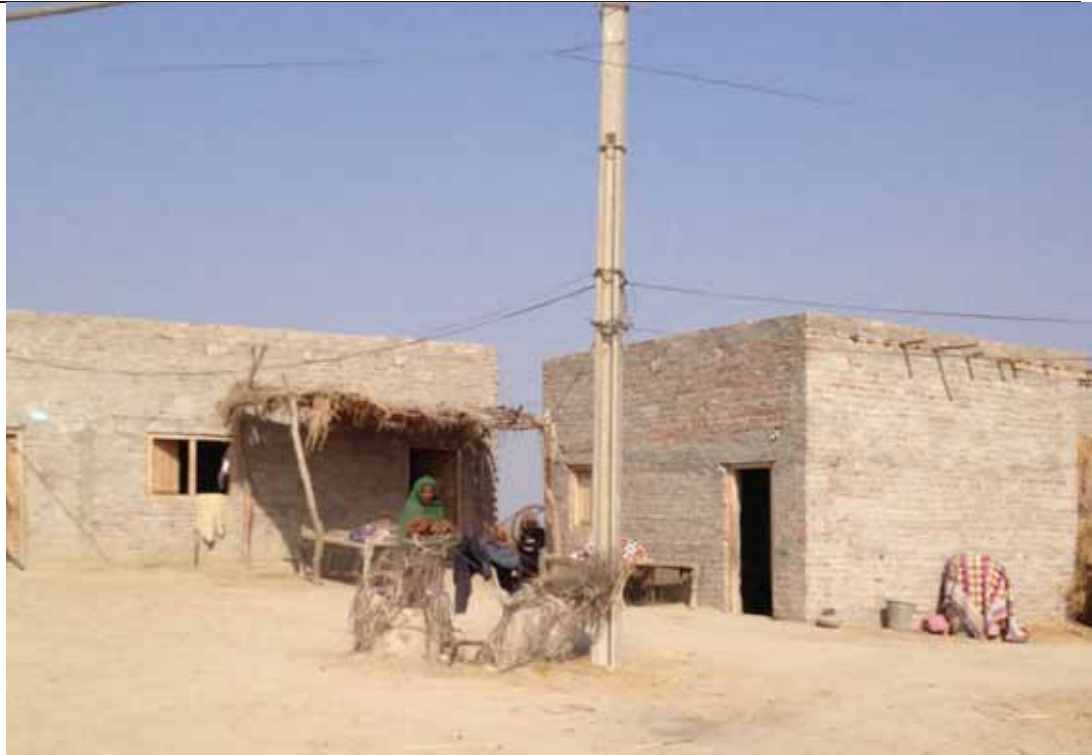
Photo 3 ACTED, Jacobabad, Pathan Khan Burnt brick ORD with flat roofs and no overhang
