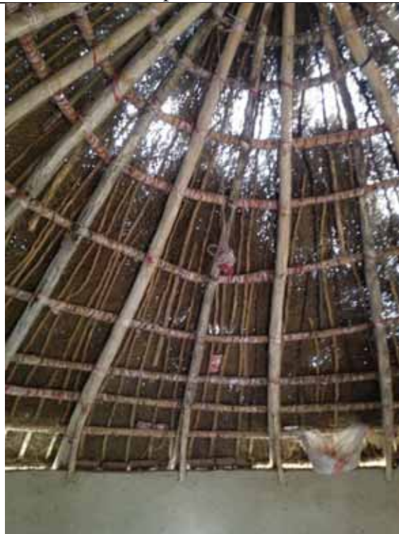
Photo 12 HANDS, Umerkot, Attar Mohammed Palliammed Palli Chora mud house with thatch roof with gaps which allow water in.
