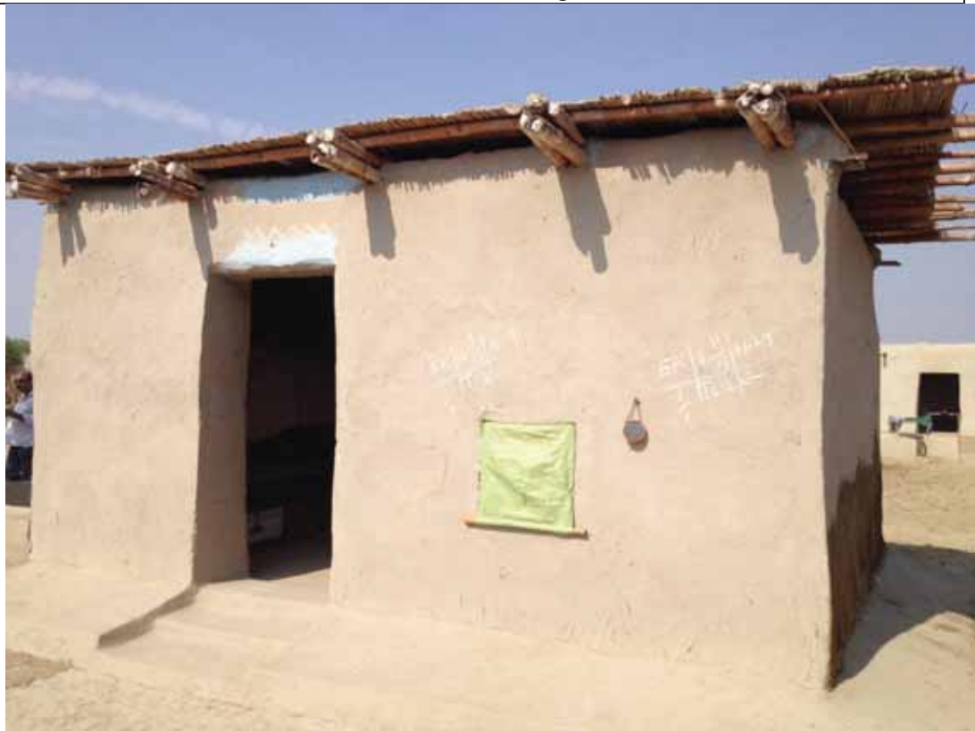
Photo 4 IOM, Umerkot, Qazi Shahid Memon Flat/ very shallow single pitch roof with small overhang
