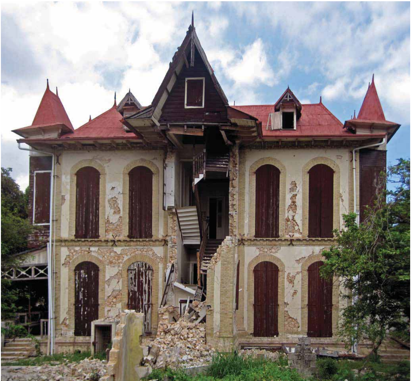
FIGURE 47 View of the back elevation of Castel Fleuri. The use of brick masonry surrounding the windows, at the corners, and at floor lines in tandem with the stucco over the stone masonry elsewhere forms a pleasing composition. Note the X-shaped end plates of the iron rods visible on the façade, which were not installed at the building corners in this case. See also Figure 108.
