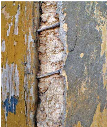
FIGURE 43 Nails help hold the earthen infill.
