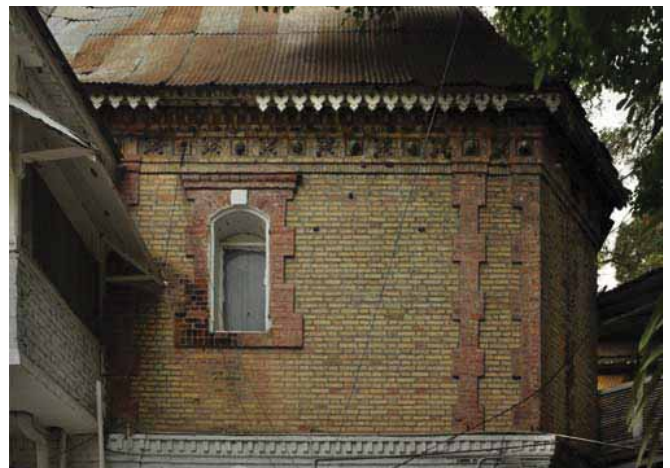
FIGURE 100 left First-floor porch of the Hotel Oloffson showing brick façade with the many door openings that surround the building on all sides. right Typical brickwork where it can be seen without the porches.
