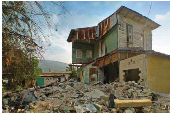
FIGURE 111 The wooden portion of this building remained standing, while the two-story concrete addition pancaked completely. This house is also shown in Figure 136 right
