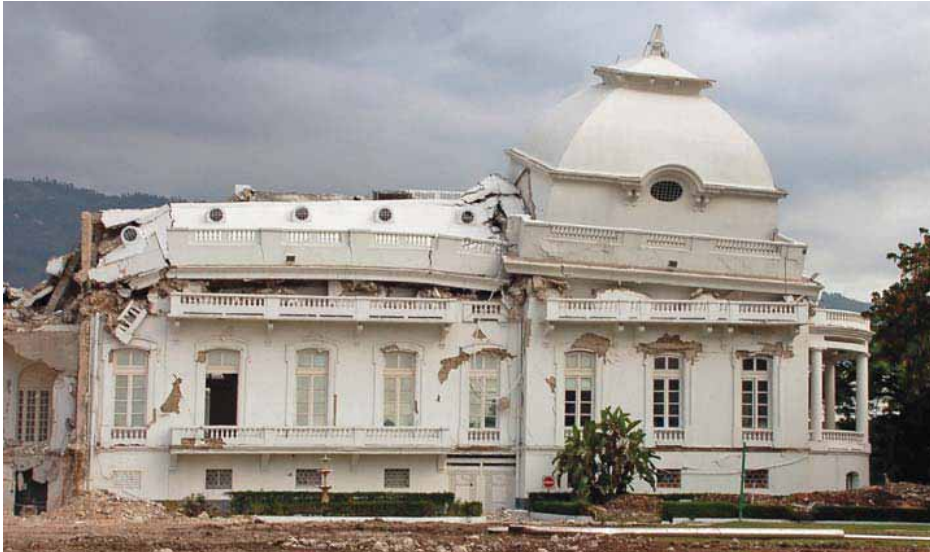
FIGURE 28 The Palais Nationale , constructed in 1918, is an example of early reinforced concrete use in Haiti. These buildings typically suffered full or partial collapse.
