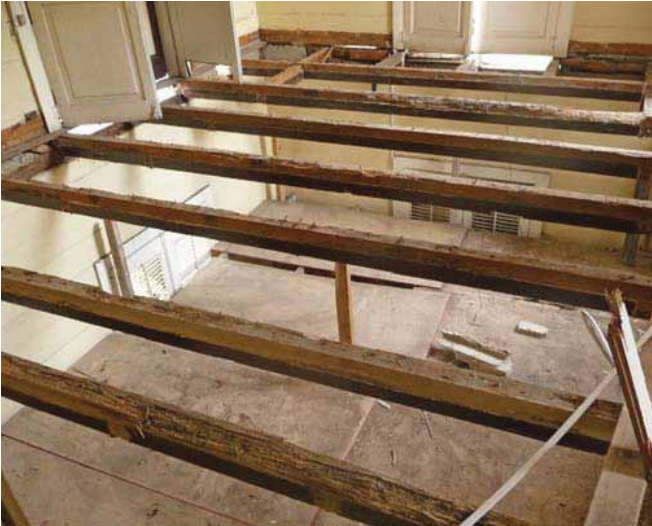
FIGURE 59 Wood floor framing with wood plank floor removed at 32 Lamartiniere.
