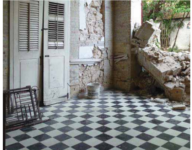
FIGURE 60 Tile over slab on grade at 5 Lavaud 1.
