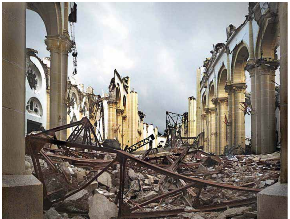
FIGURE 131: interior of the Cathédrale Notre Dame de L'Assomption after the 2010 earthquake suffered a complete roof collapse, collapse of sections of its interior arcades, and collapse of the tops of its two bell towers. Remarkably, all four of its two-story exterior facades remained largely intact. The building was constructed between 1884 and 1914, with walls of reinforced concrete with infill masonry construction. Much of the reinforcing had become heavily corroded by the time of the earthquake. Weak bonding due to the use of smooth rebar also made this and other reinforced concrete structures particularly vulnerable to seismic damage.
