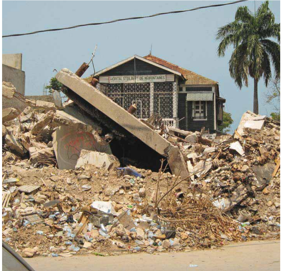
FIGURE 118 In a typical scene, a Gingerbread stands intact beyond the tragic collapse of a modern concrete building
