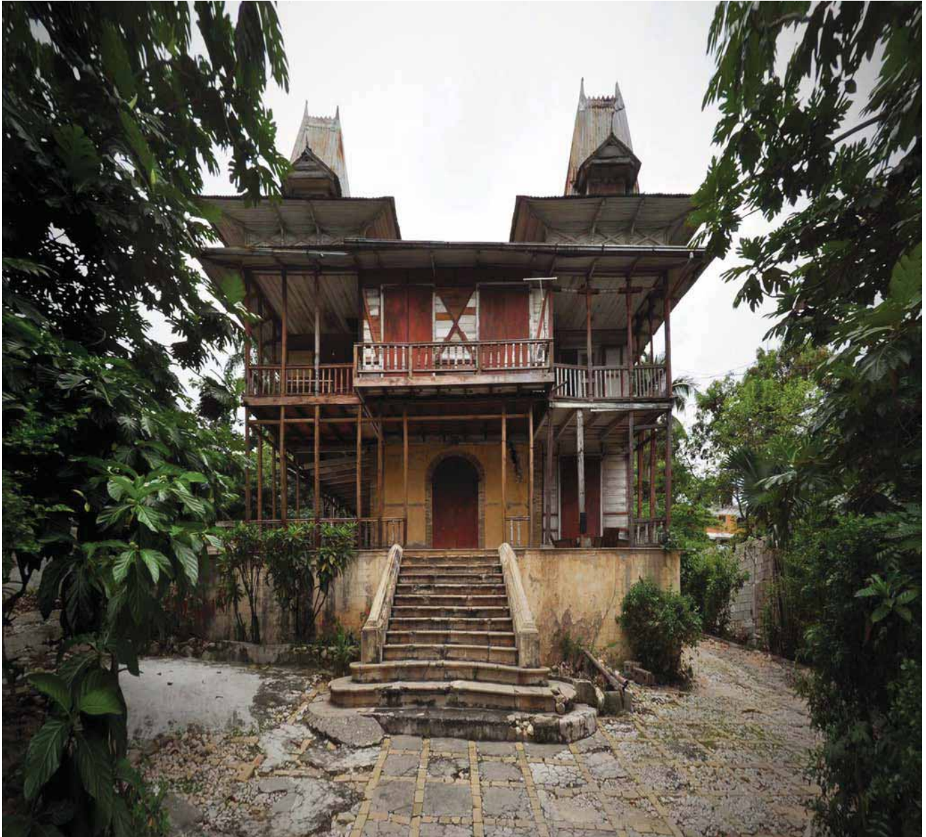
FIGURE 1 cover: The west front of the Villa Castel Fleuri on Avenue Christophe, a grand brick and rubble stone masonry house. This house was occupied by the President of Haiti for a short period in its history. It has suffered extensive damage in the earthquake mainly to the projecting stair tower on the east side, and porches on the west. The plates that hold the iron ties that penetrate the building are visible on the façade.
