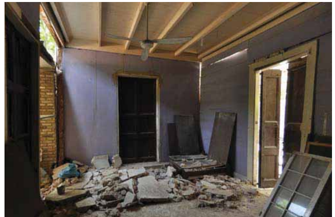
FIGURE 73 These are examples of colomage where the rubble infill has been replaced with concrete. This has accelerated the rotting of the timber framing, which then broke during the earthquake causing the collapse of the heavy concrete infill.
