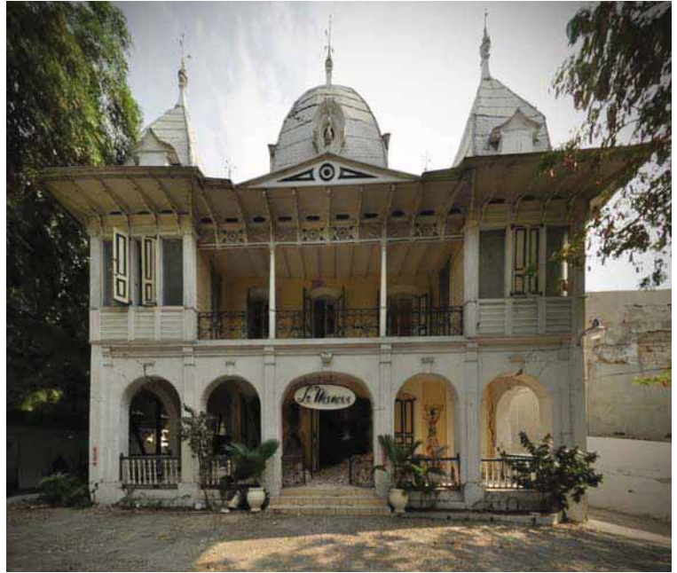
FIGURE 96 top Exterior view of Le Manoir on Avenue John Brown. middle interior view of Le Manoir showing a fully disrupted ground-floor wall where the rubble panels have collapsed, but the buildings remained standing on the brick piers. (view is a mosaic of several photos connected together). bottom House at 65 Avenue N showing infill panels manifesting the onset of damage, but little displacement during the earthquake.
