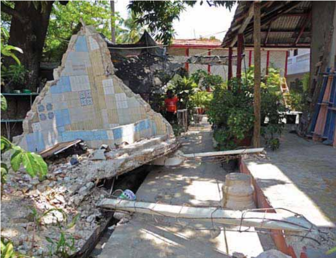
FIGURE 70 This second floor concrete bathroom addition at 5 Lamartiniere landed on the ground after its concrete columns buckled as it pulled away from its parent Gingerbread house. Note sewer pipes in the center of the rebar of the buckled columns.
