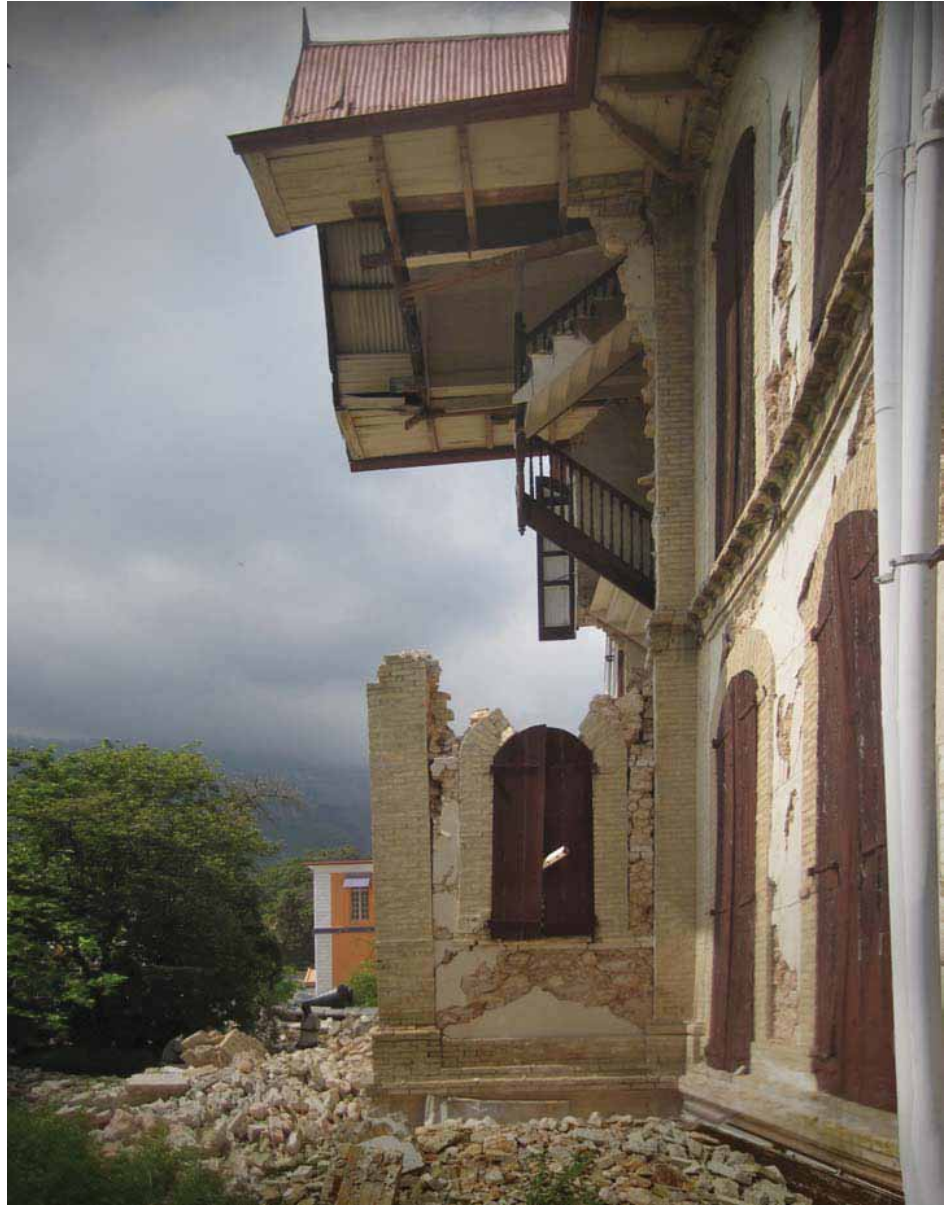
FIGURE 129 The collapsed rear entrance of the Villa Castel Fleuri on Avenue Christophe, which suffered extensive damage in the earthquake.
