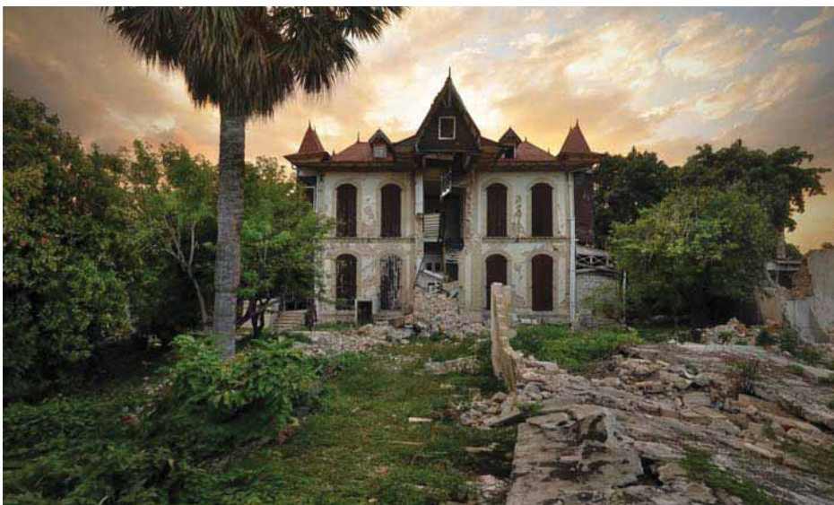
FIGURE 29 The east (back) elevation of the Villa Castel Fleuri on Avenue Christophe, a grand brick and rubble stone masonry house. This house was occupied by the President of Haiti for a short period in its history. It has suffered extensive damage in the earthquake mainly to the projecting stair tower on the east side, and porches on the west. The plates that hold the iron ties that penetrate the building are visible on the façade. See also Figure 47 on page 29.
