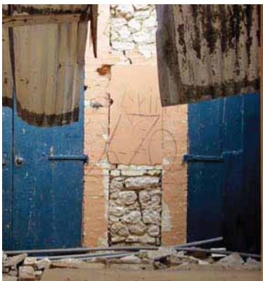
FIGURE 46 Characteristic 'brick frame' with rubble infill construction
