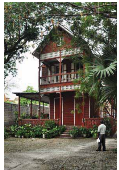
FIGURE 35 24 Avenue Lamartiniere, the wood-frame house also shown in Figure 34.
