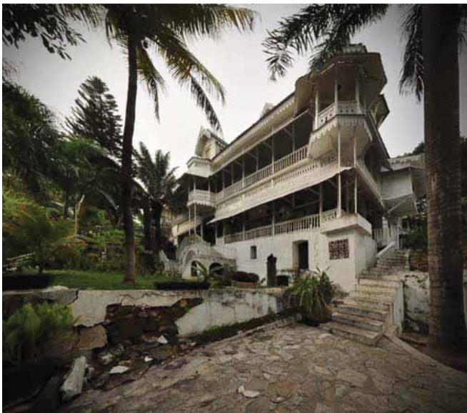
FIGURE 99 The Hotel Oloffson. This building is constructed of brick masonry without the rubble stone panels. The masonry walls are hidden in the front by the wide wooden Gingerbread-clad porches, but are visible below.
