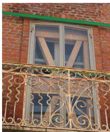
FIGURE 138 Examples of shoring constructed after the two recent earthquakes in Italy demonstrate different solutions to the important problem of stabilizing heritage structures to avoid emergency demolition for public safety. The two photos on this page show an unreinforced masonry building damaged in the 2002 Molise earthquake shored entirely with polyester straps, thus eliminating the need to block the street with diagonal braces. Shoring has been installed in the window openings—an important part of any system as it gives the damaged masonry wall structural continuity across openings.
