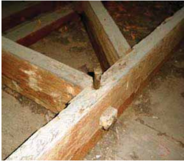
FIGURE 53 Attic framing with mortise-and-tenon joinery with wooden peg.
