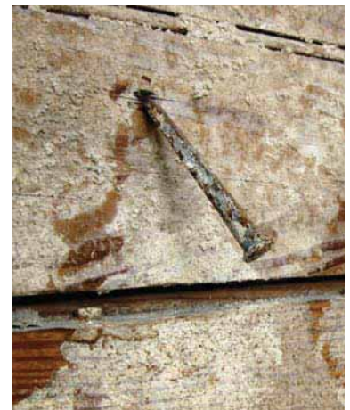
FIGURE 81 Cut nails of iron or steel are common in the Gingerbread houses. Many of the original cut nails show surprisingly little corrosion.
