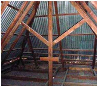
FIGURE 54 Corrugated steel roof over purlins and braced roof framing.
