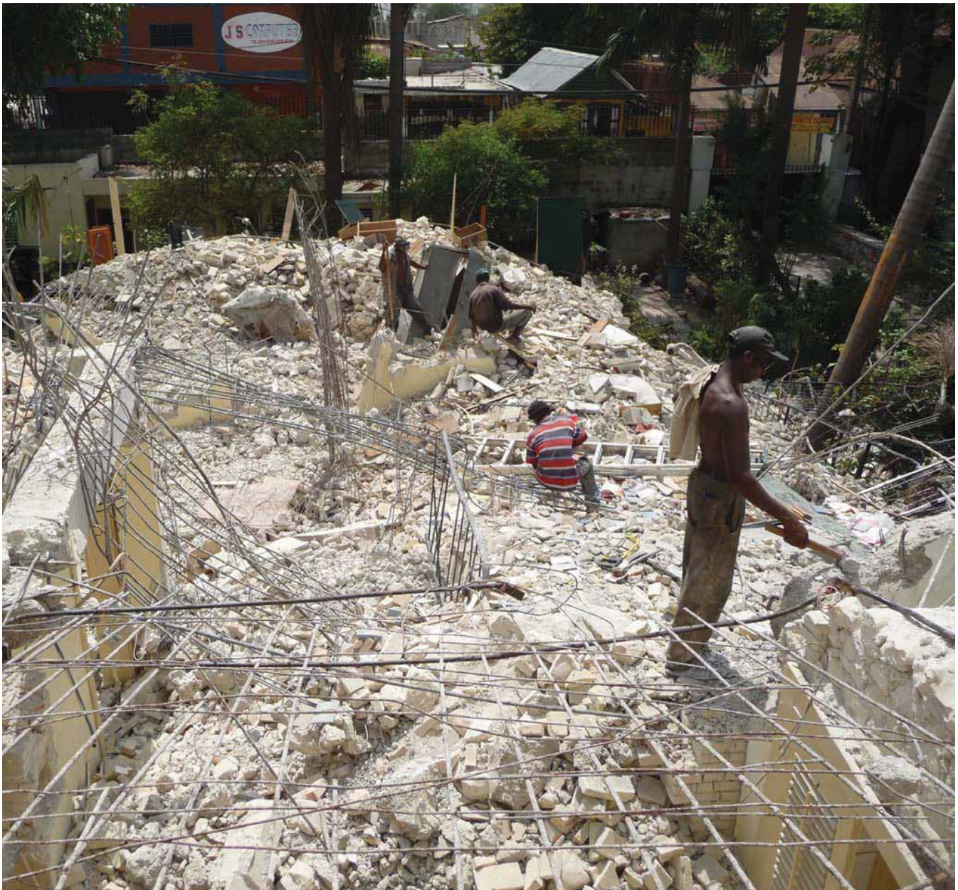
FIGURE 117 Demolition of a collapsed reinforced concrete building using small sledge hammers.
