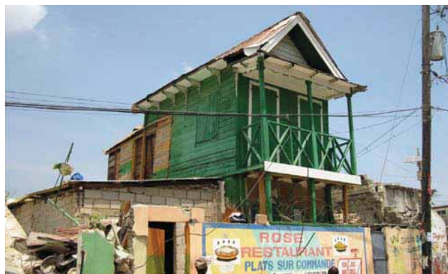
FIGURE 76 This two-story Gingerbread house survived amid the collapse of numerous concrete buildings. The owners do not want to tear it down. However, it needs temporary stabilization and long-term repairs.
