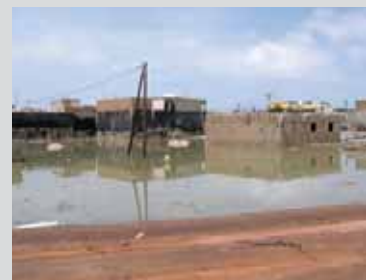
Floods in urban areas of Saint Louis in Senegal
