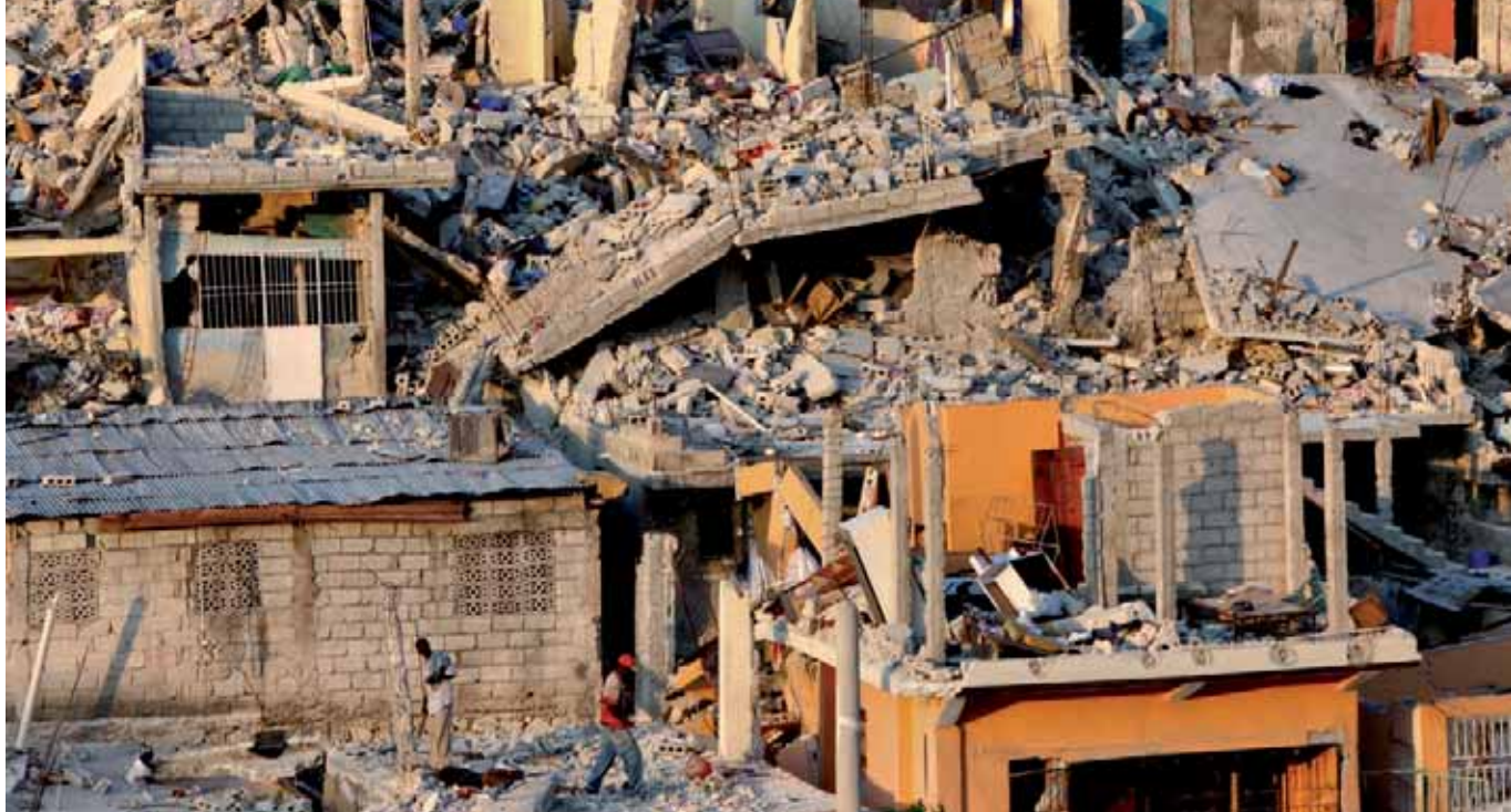
Severe damages after the Haiti earthquake (2010) Marco Kokic (ICRC)
