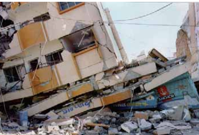
Earthquake damage in Bhuj, India (2001)
