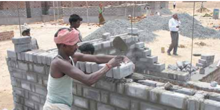
'Rat-trap bond' masonry Skat
