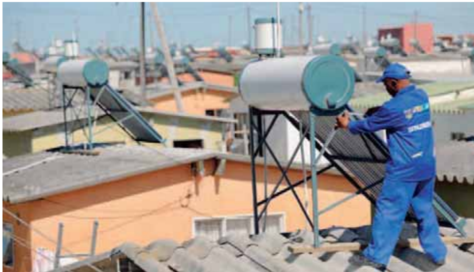
Solar panels for hot-water production in Bruce Sutherland, City of Cape Town 61
