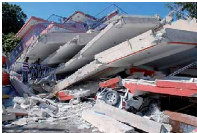
Earthquake damage in Haiti (2010)
