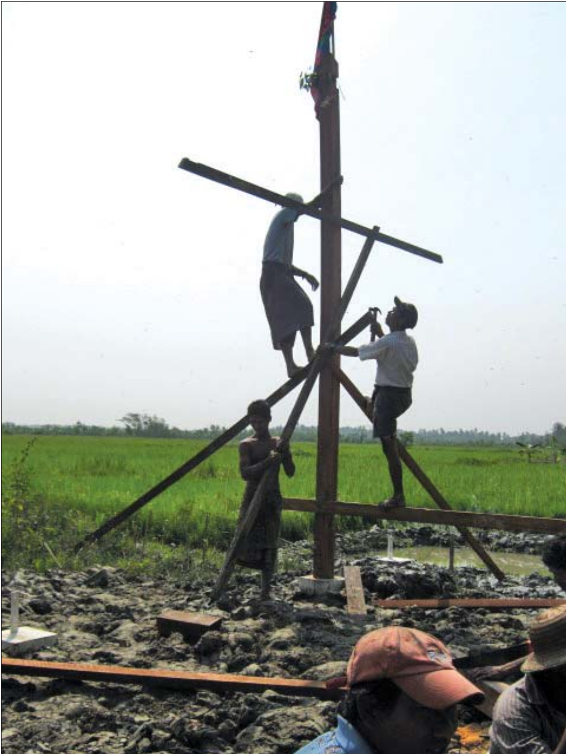
Posts held in position with temporary supports ▲
