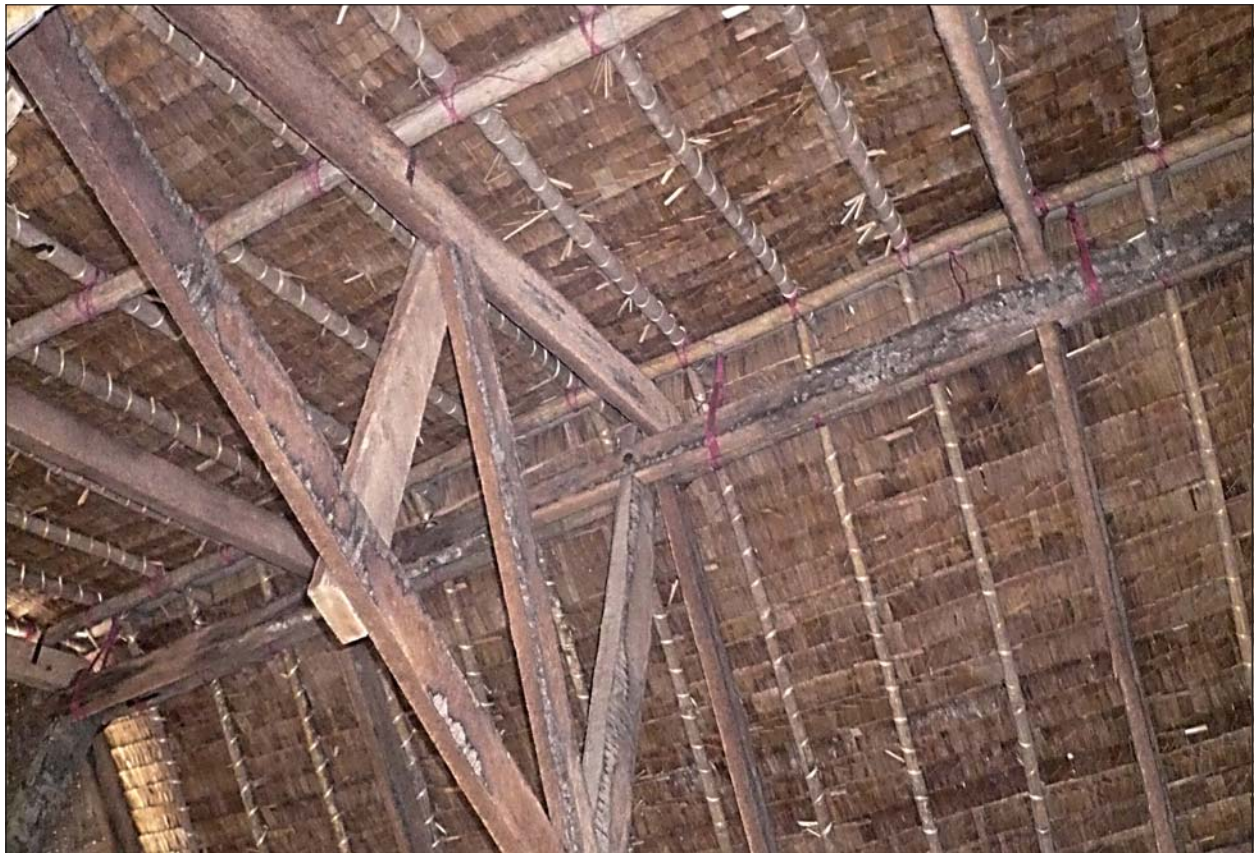
"Dani" roof viewed from inside ▲
