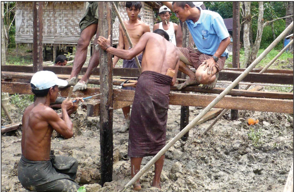
Fixing floor joists ▲
