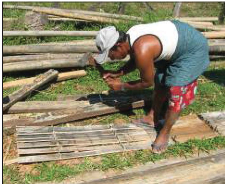
◀ Preparing a bamboo floor mat
