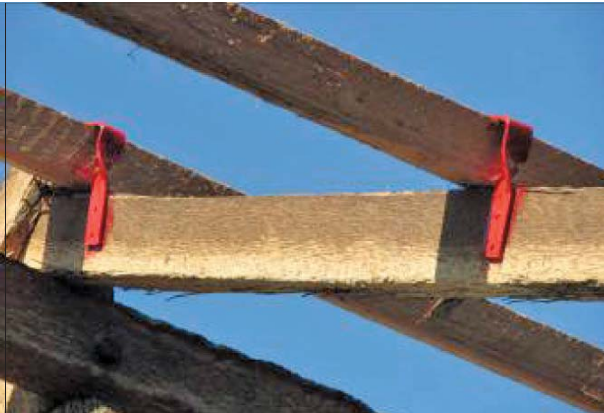
Steel straps to anchor runners to rafters ▲
