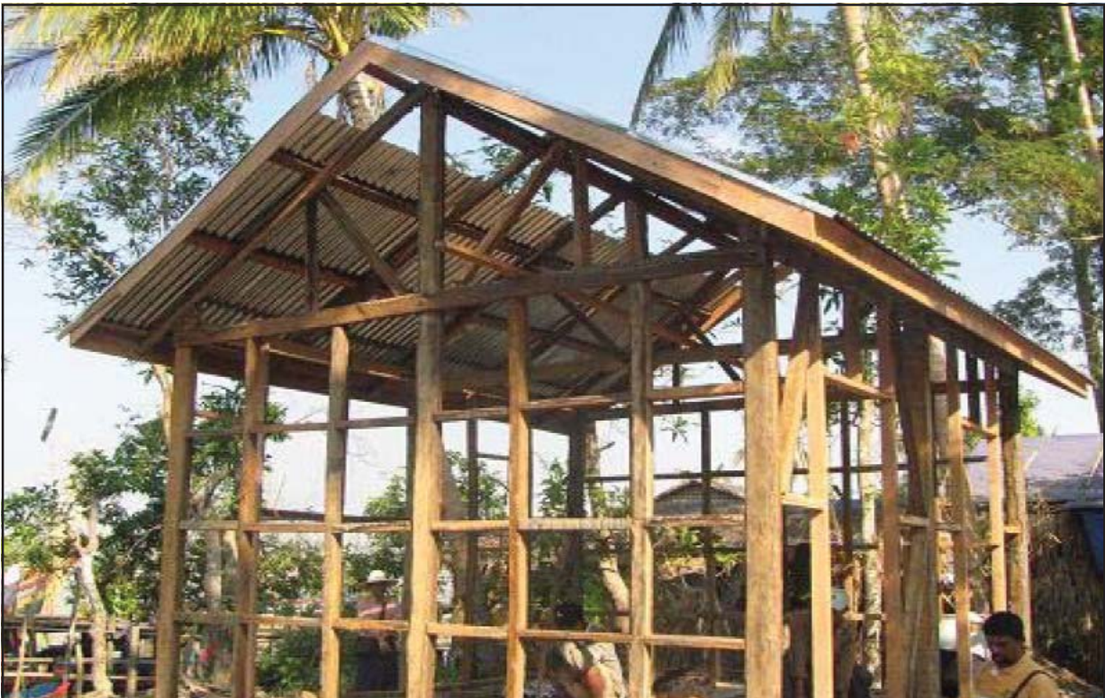
Framework for wall cladding ▲
