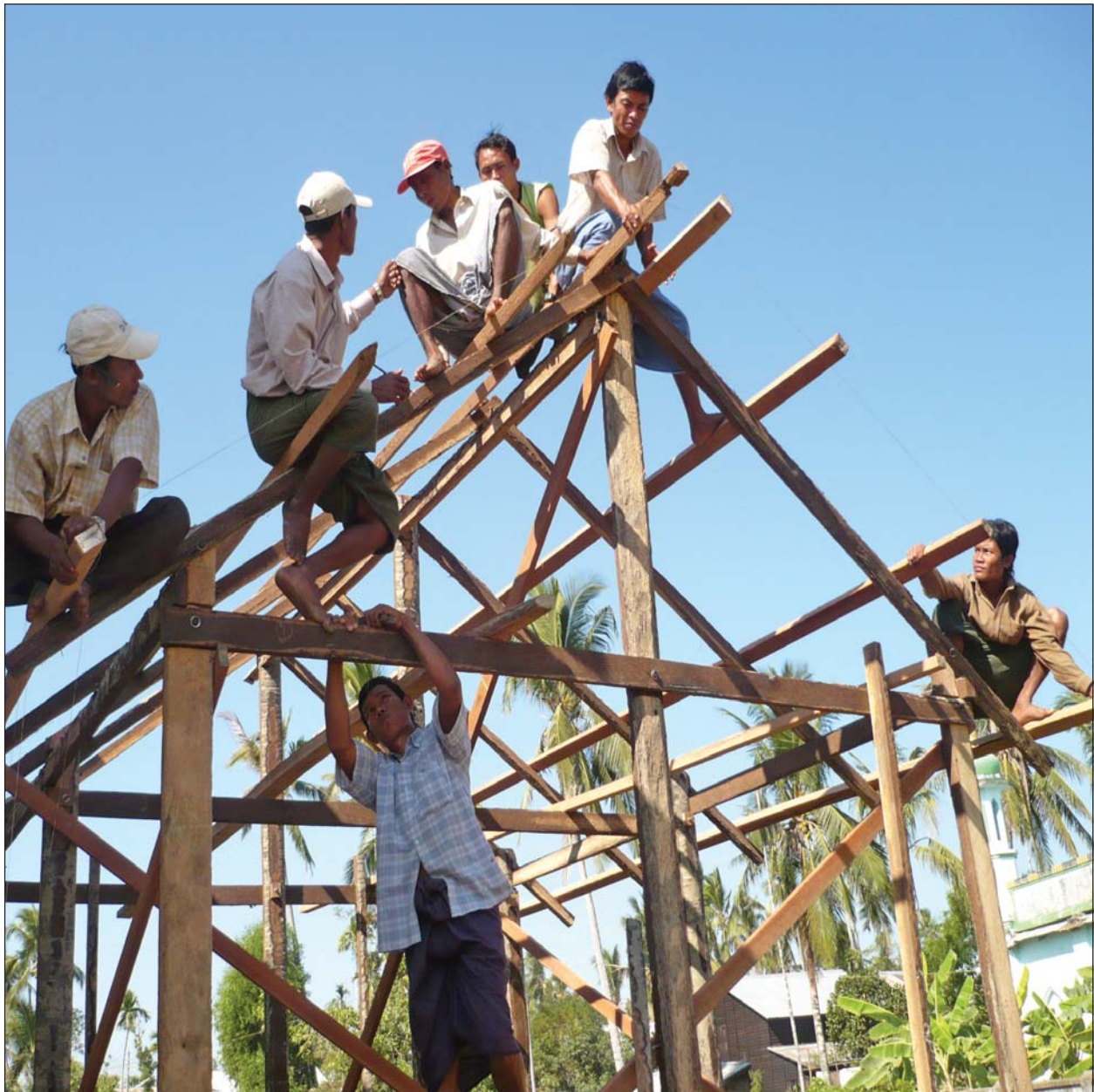
Pair of rafters being erected ▲
