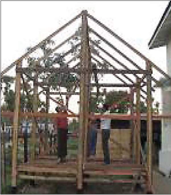
All rafters in position ▲
