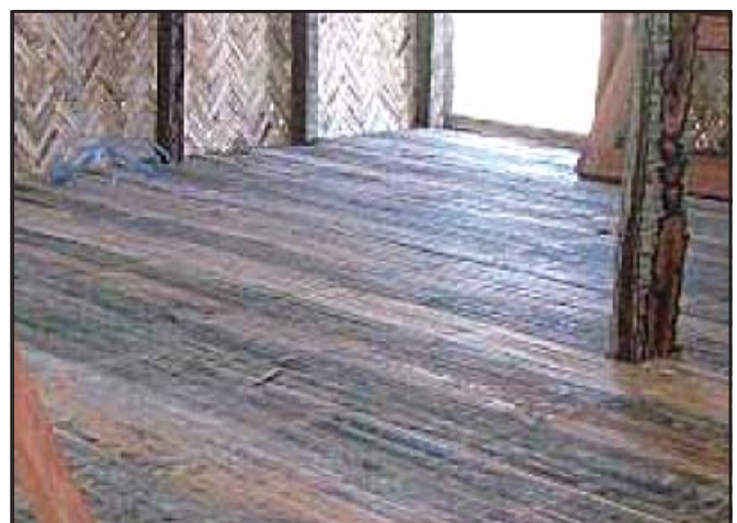
House with Bamboo floor mat ➤
