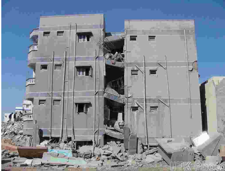
Collapse of open ground storey RC frame residential building in Bhuj.
