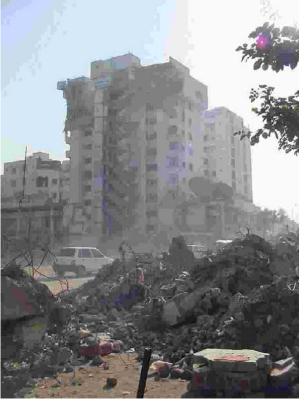
Collapse of one-half of the 14-storey RC frame residential apartment building in Ahmedabad; the collapsed portion had a swimming pool on the roof, unlike the other half that is standing.
