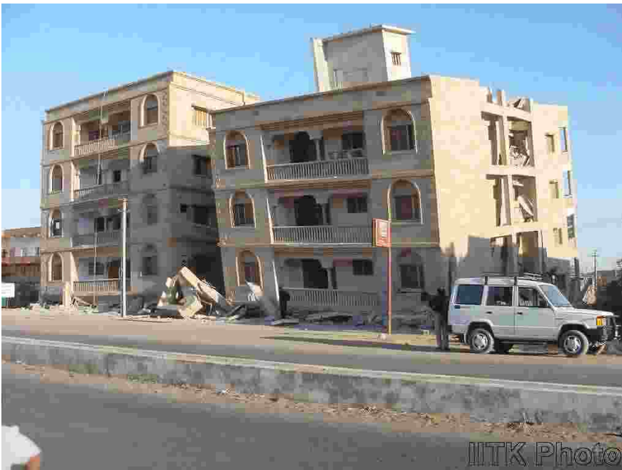
Ground storey collapse of a 4-storey building with open ground storey at Bhuj.
