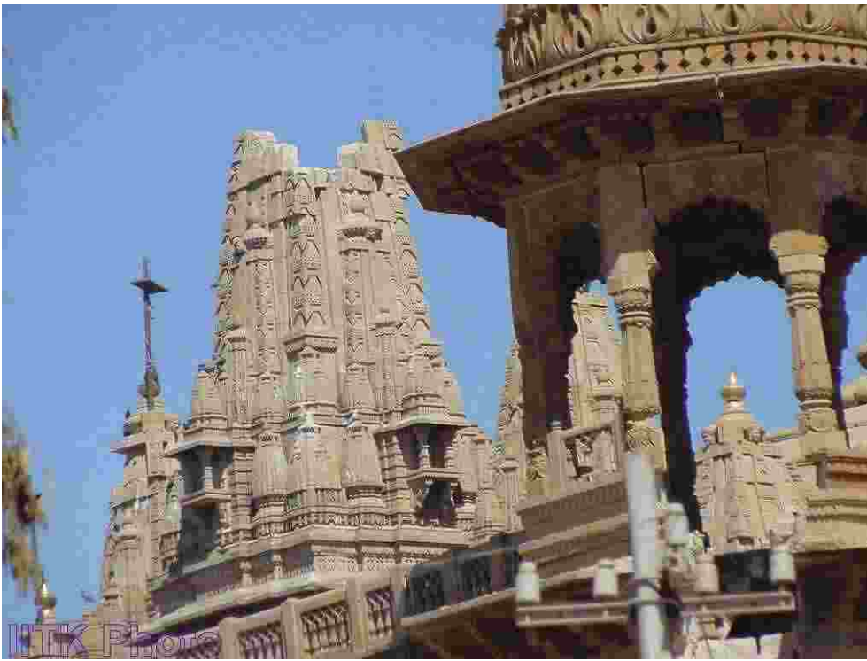
Partially collapsed pagoda at the palace at Morbi.
