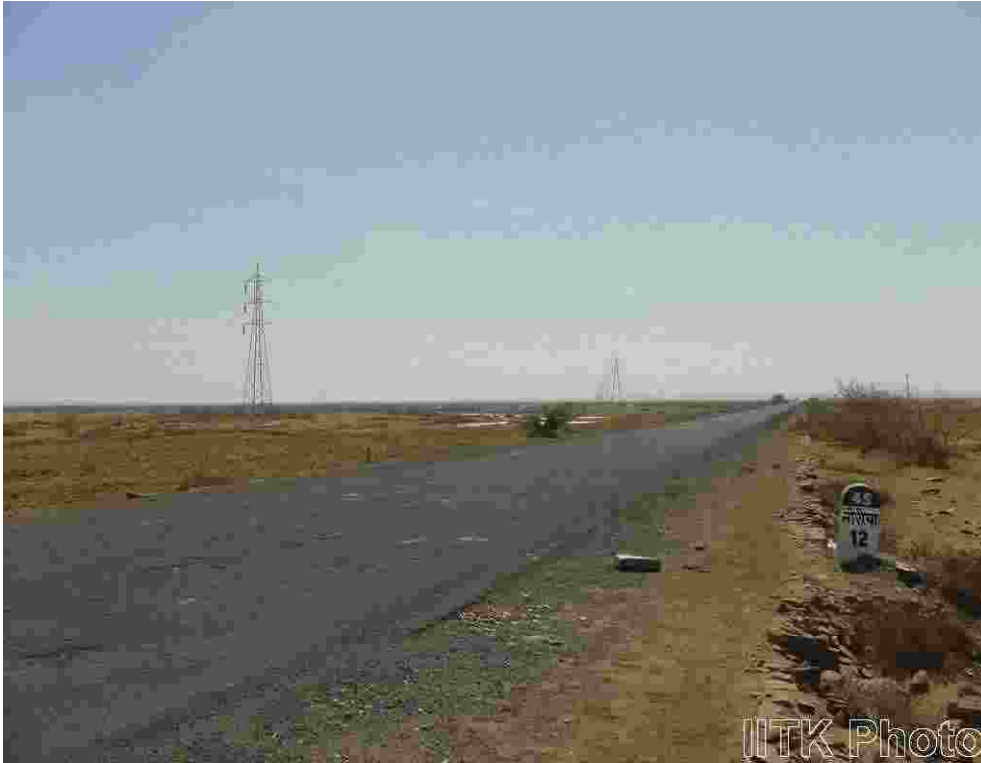
Steel HT lines near Khawda and elsewhere did well during the earthquake.
