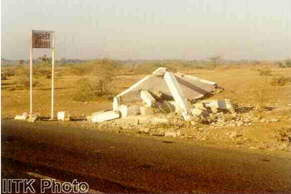
Collapse of the RC frame shelter at a bus stop near Pundi village.
