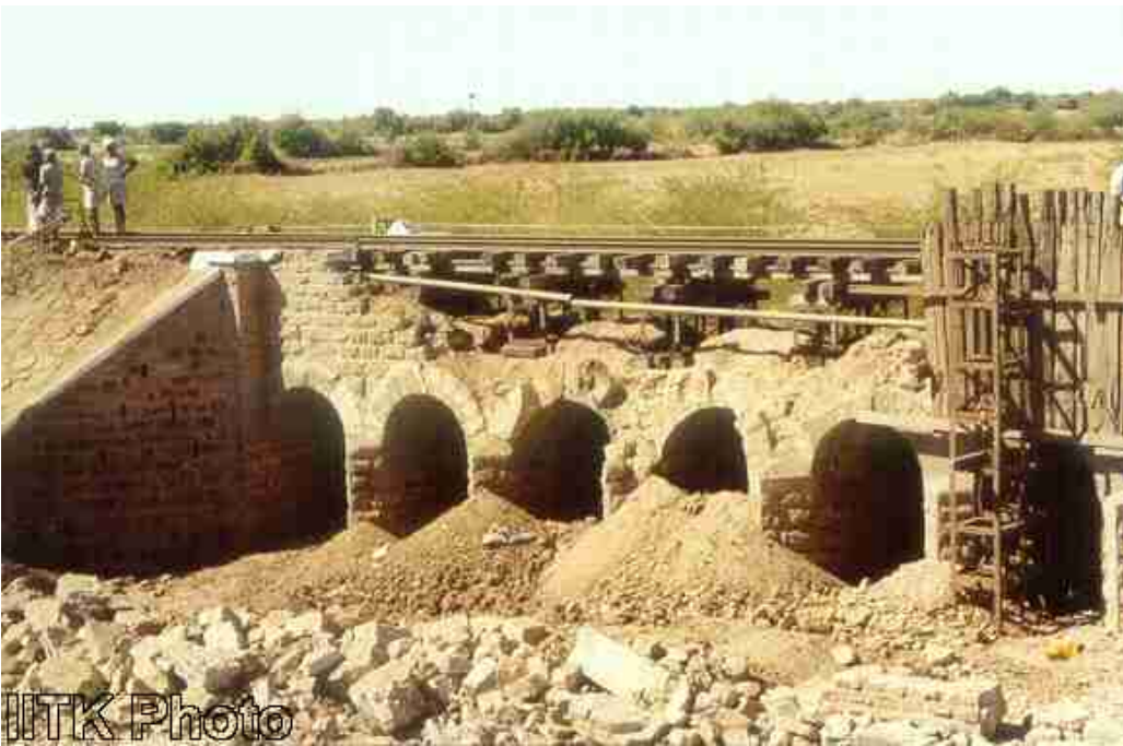
A number of old masonry arch bridges for Indian railways sustained extensive damage. This bridge is about 88 years old.
