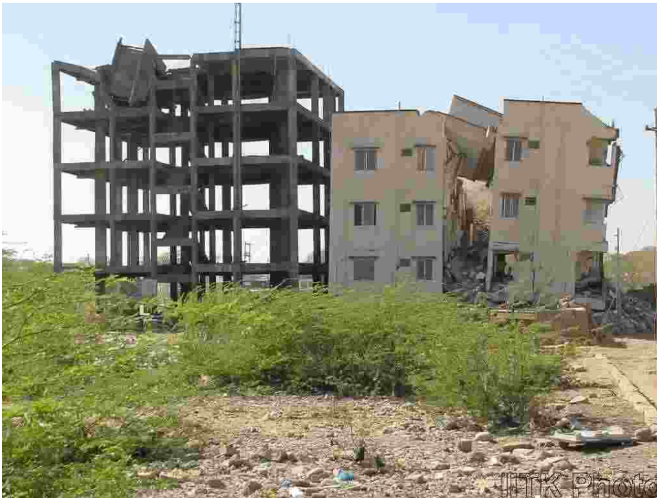
Numerous cases of dislodging of the weakly connected overhead storage water tanks were observed in the entire earthquake affected area. Picture shows dislodging of water tank appendages from atop unfinished and finished RC frame buildings in Bhuj.
