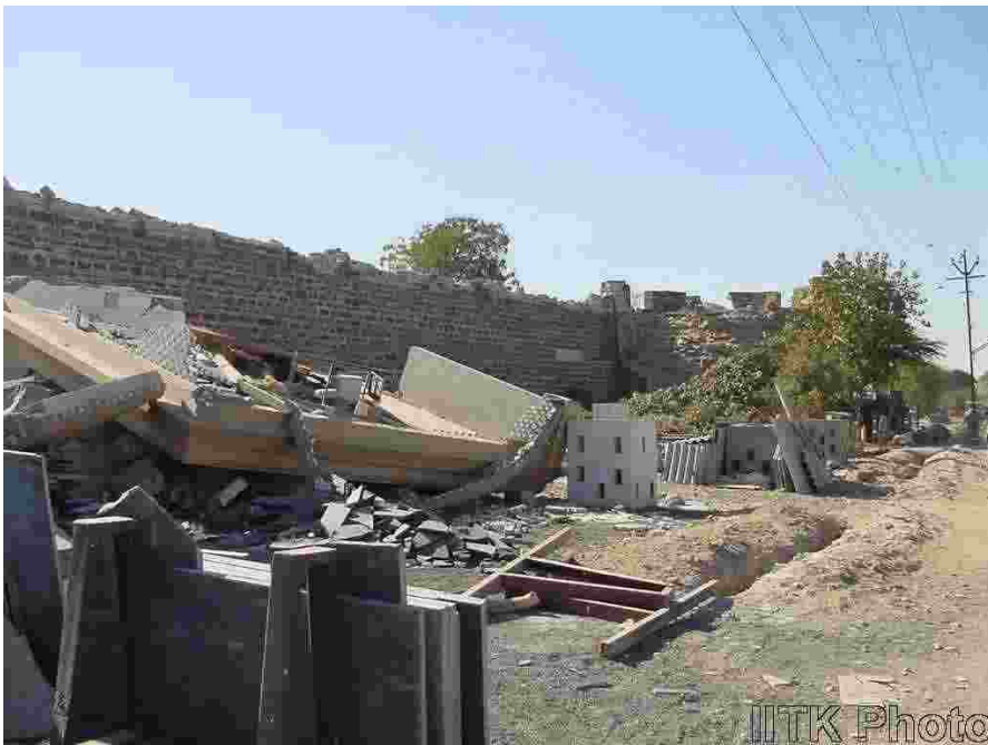
Partial collapse of the walls of the historic fort at Bhuj.
