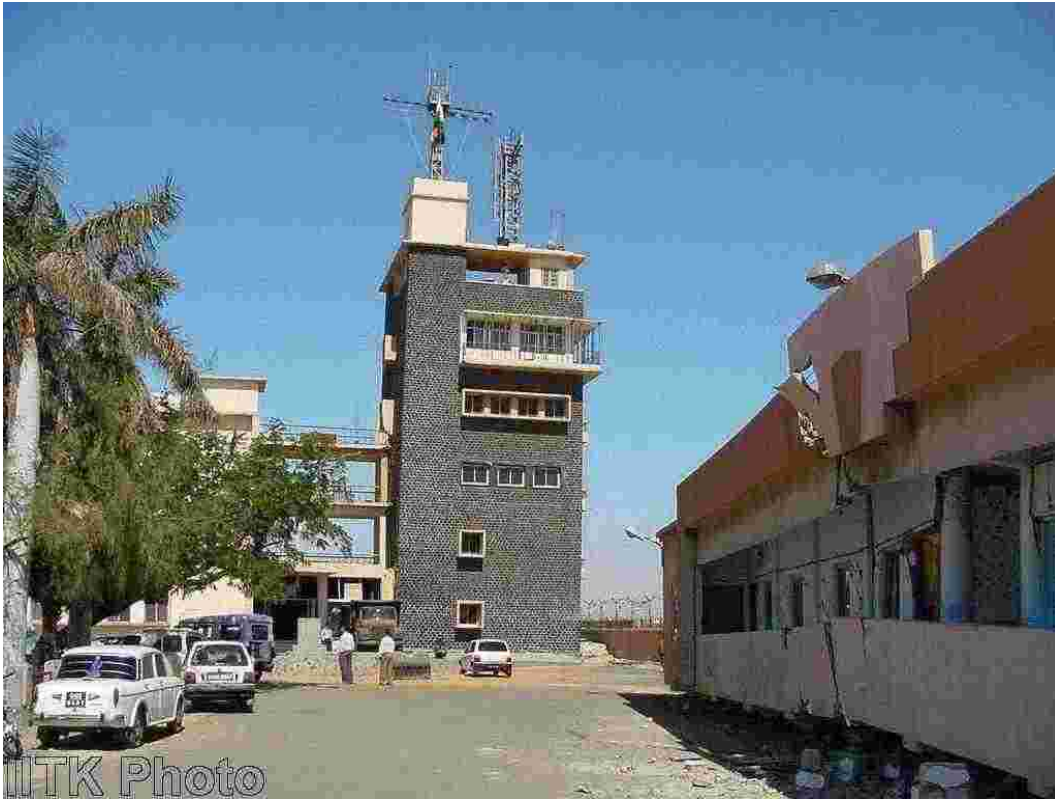
A 15° tilt in the 6-storey control tower at Kandla port due to liquefaction and consequent lateral spreading towards the bay.
