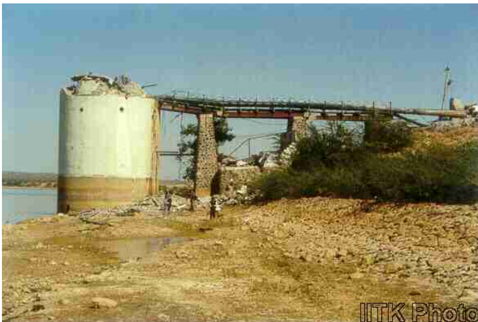
Collapse of the random rubble masonry intake tower at the Tappar Dam.
