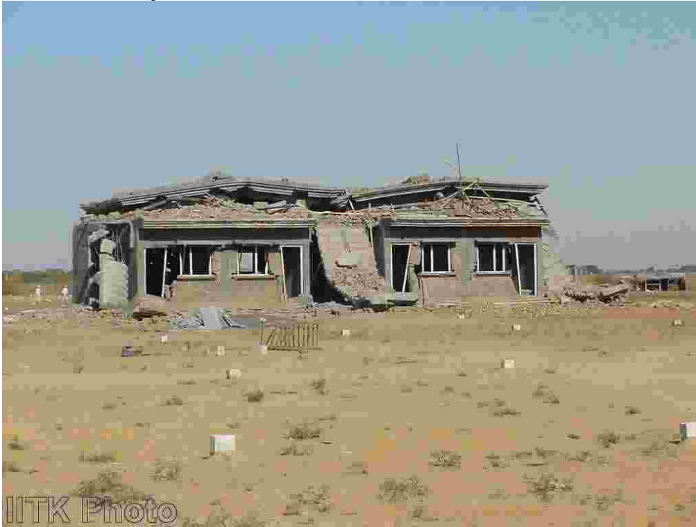
Collapse of the upper storey of a building under construction at Bhachau village.
