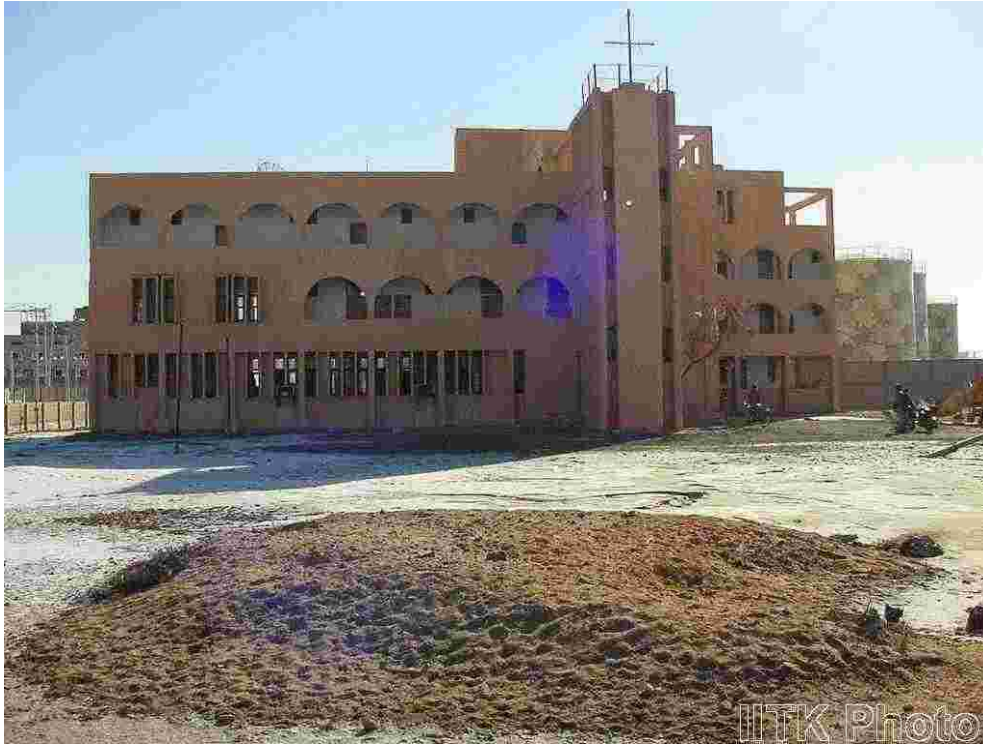
Extensive liquefaction near a 3-storey RC frame office building at Kandla port; building sustained only minor cracks in the walls, but settled down by about 70mm.
