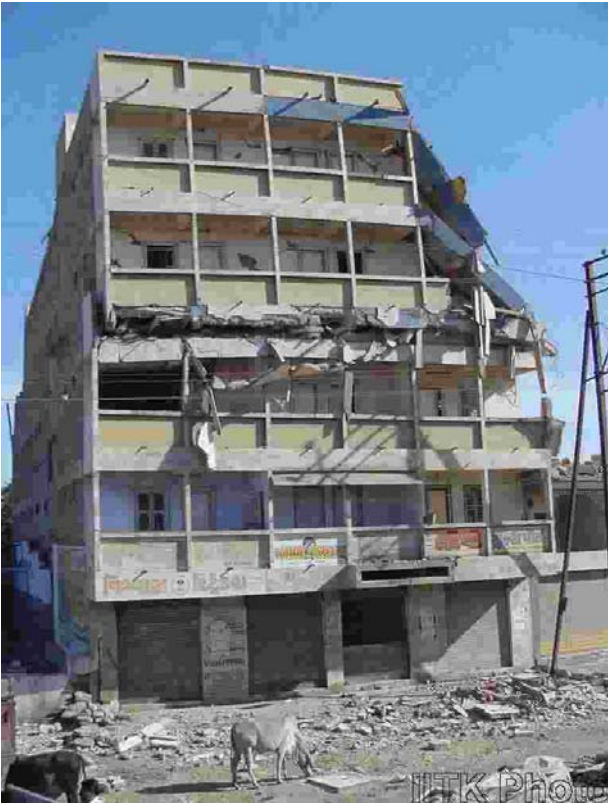
Collapse of intermediate storey in a 6-storey RC frame commercial building at Bhuj.
