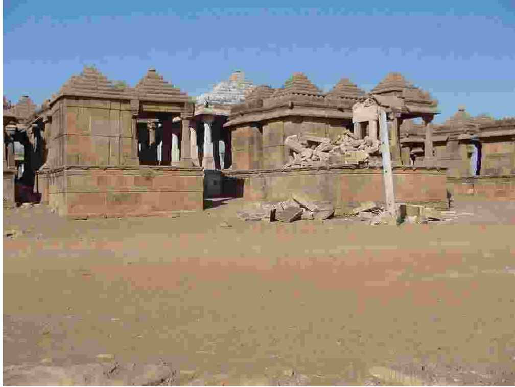
Collapse of the temple pagodas made of large block stone masonry at Halvad near Ahmedabad.
