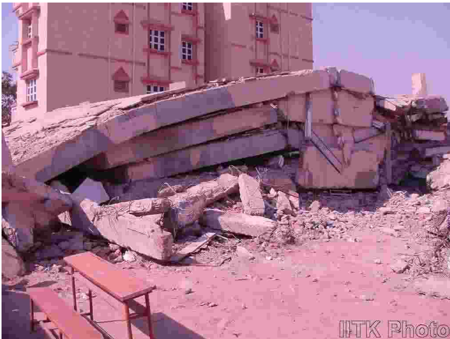
Pancake collapse of 4-storey L-shaped RC framed school building in Ahmedabad.
