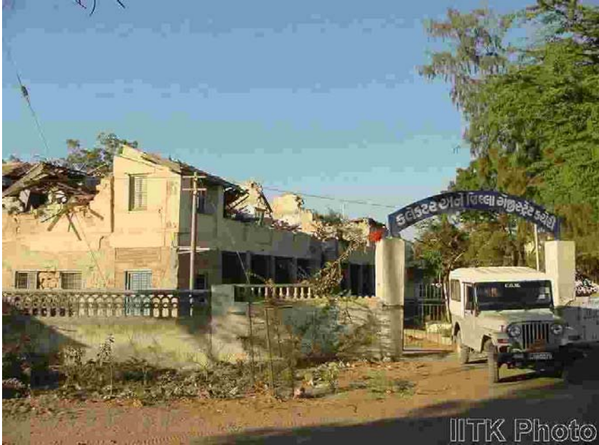
Collapse of the upper storey of the block masonry government office building at Bhuj.
