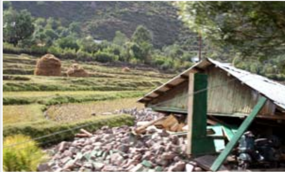
The damage of the buildings in the Uri area after the earthquake varied and was categorised by AIDMI in total, partial and internal collapse.
