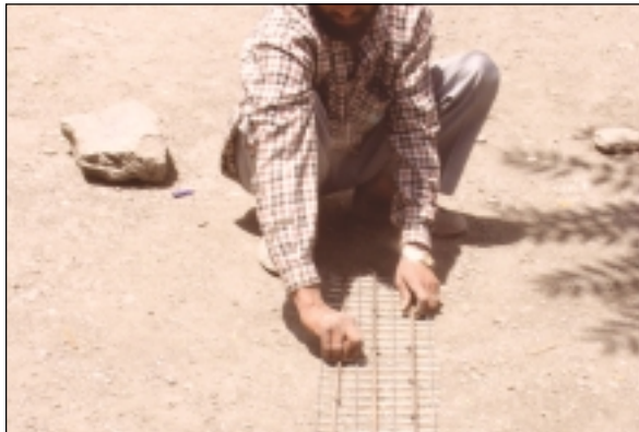
Preparing WWM with 6 mm rebars
