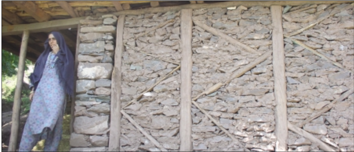
Dhajji wall with inadequate bracing & strut system
