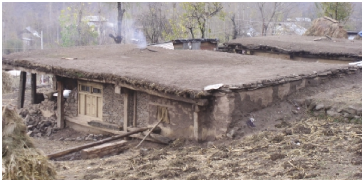
Traditional flat mud roof on timber understructure with stone masonry walls
