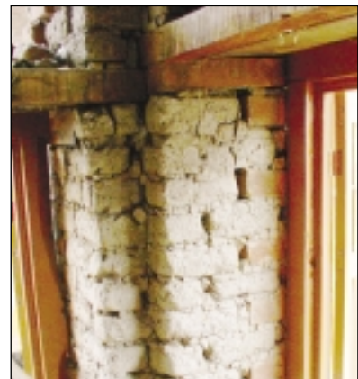
Unbaked brick with baked brick veneer
