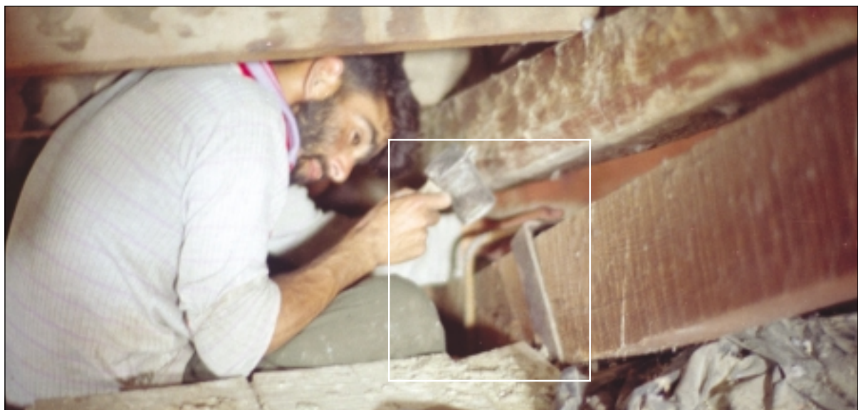
Anchoring Roof truss to wall with 'U' clamp
