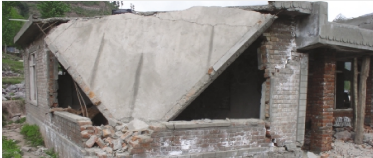
Partially collapsed RCC roof
