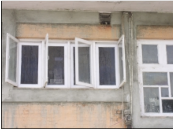
Encasement of windows
