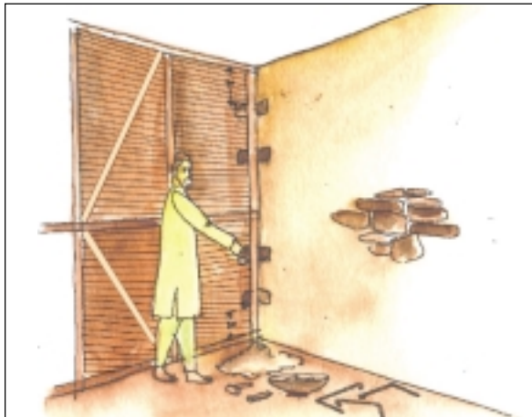
Making holes for anchors in adjacent walls
