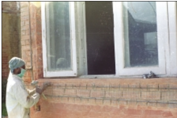
Installing WWM with bars to walls
