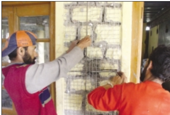
Tying encasement reinforcement to shear connector dowel
