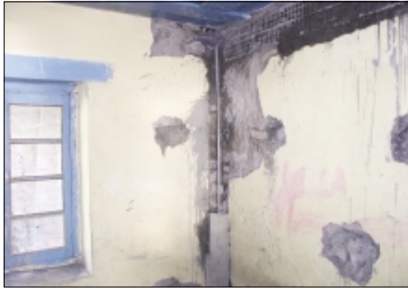
Installing vertical reinforcement in the corner
