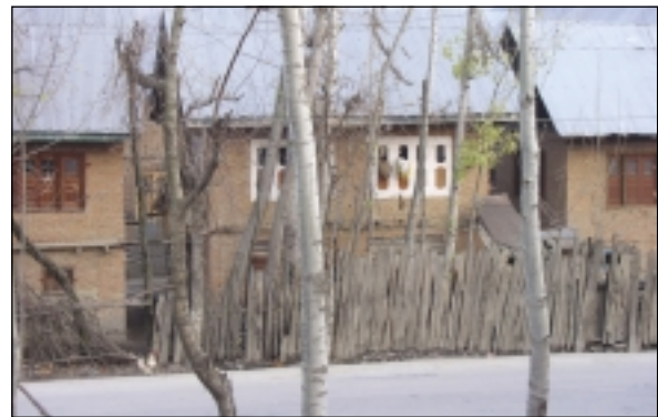
CGI sheet roofing on timber and burnt brick masonry wall
