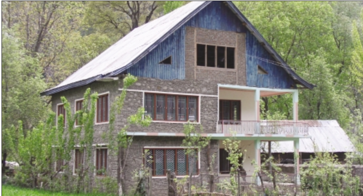
Typical house with random rubble wall & CGI roof
