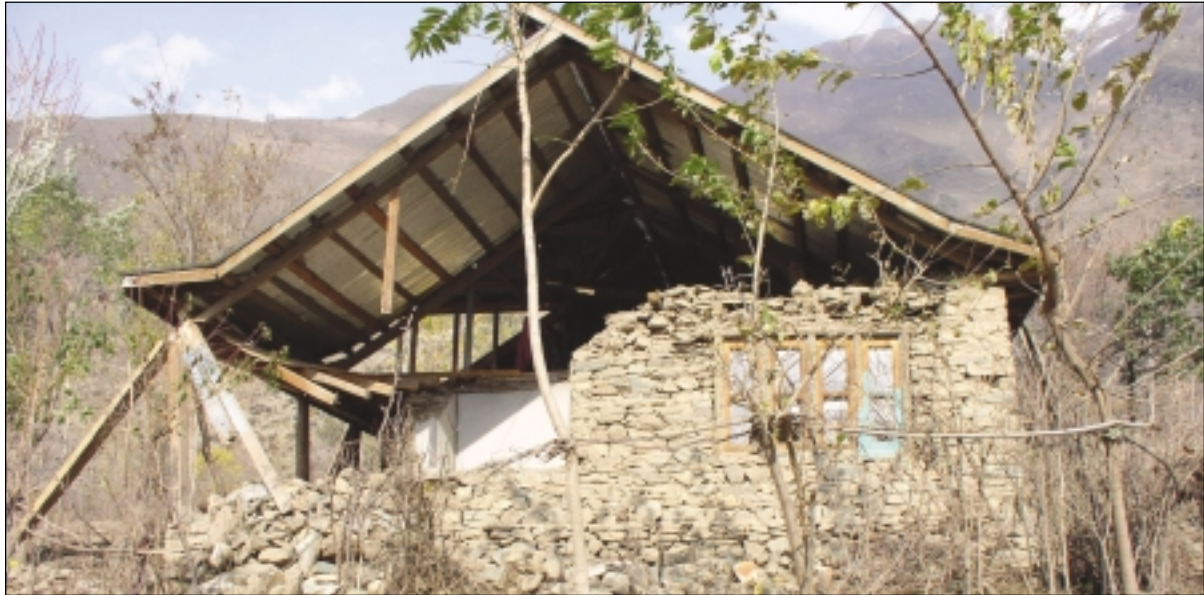
Roof damaged due to inadequate tying
