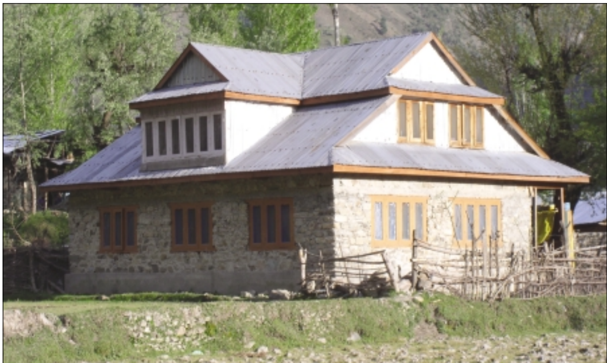
Four sided CGI roof on random rubble walls
