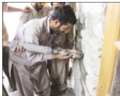
Grouting no-shrink grout in crack with hand pump
