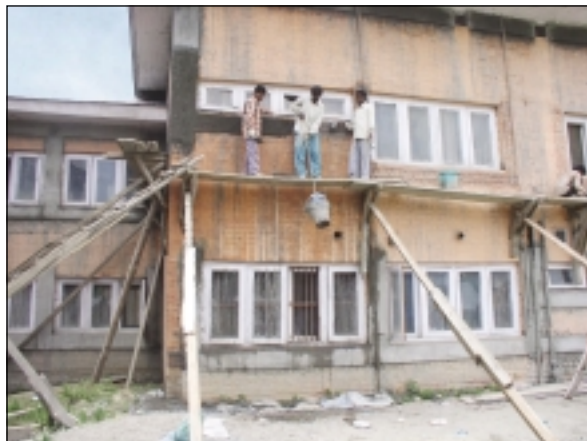
Retrofitting work in progress
