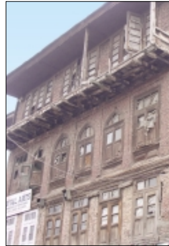
Taaq type construction
