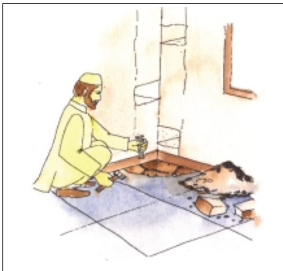
Breaking flooring and digging hole for vertical bar anchor
