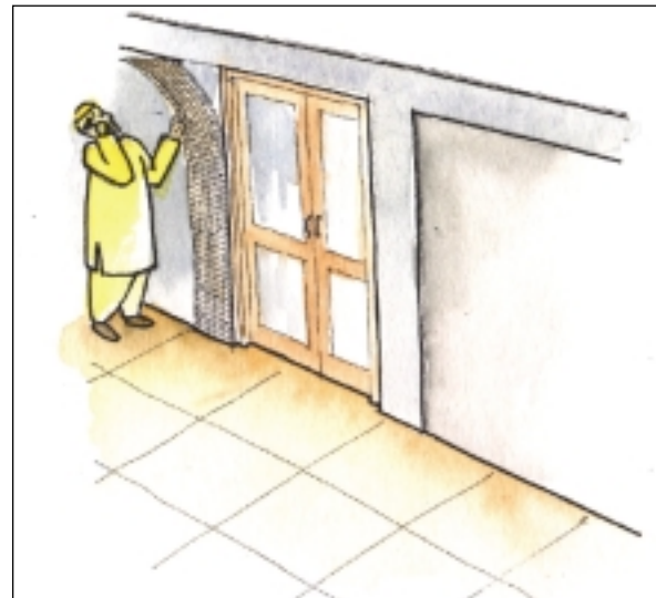
Installing WWM around door opening
