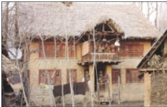
Thatch roofing on timber and burnt brick masonry wall
