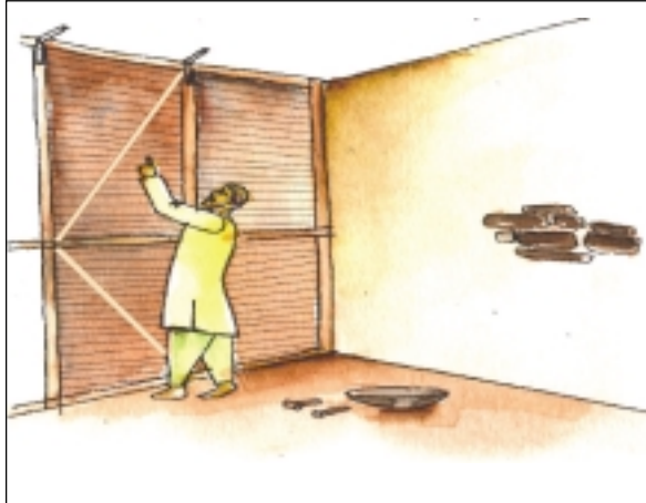
Anchoring Dhajji wall to roof deck
