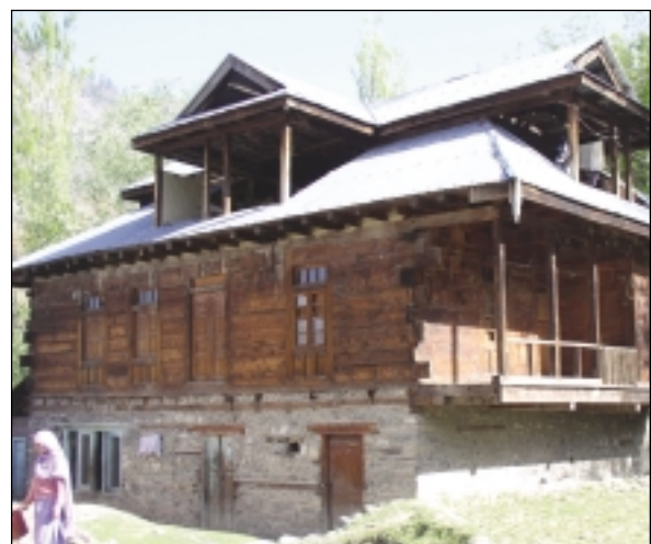
Four-sided CGI roof on timber and random rubble walls
