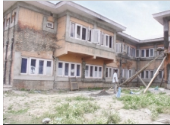
Eave-level belt and opening encasement
