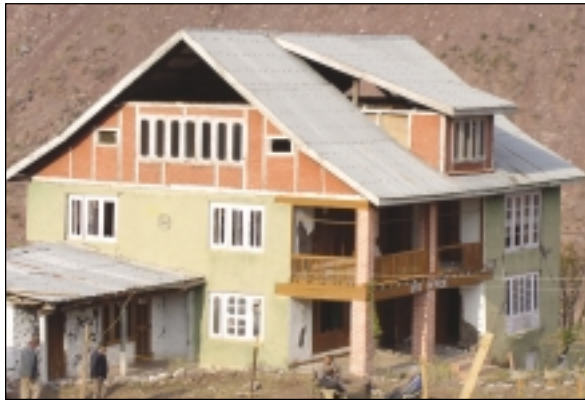
Burnt and unburnt brick masonry walls with CGI roofing on timber
