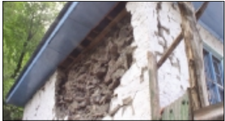
Delaminated wall
