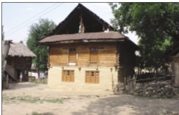
CGI sheet roofing on stone masonry and timber wall
