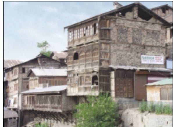
House with timber balconies and two sided pitched roof
