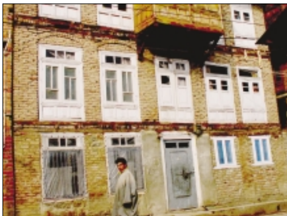
Taaq type construction
