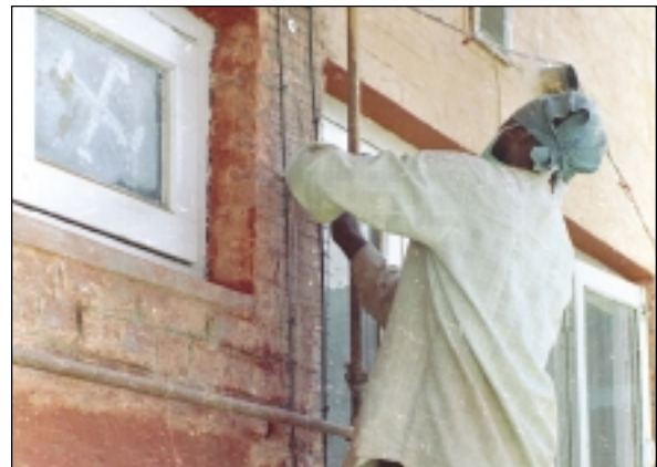
Installing WWM with bars on the walls
