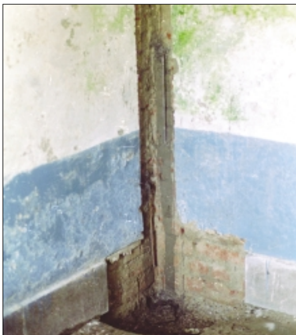
Installing vertical reinforcement at inside corners
