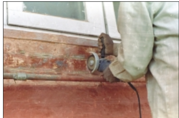
Raking mortar joints with power grinder
