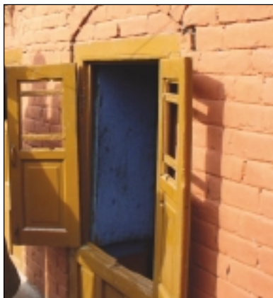
Baked brick wall
