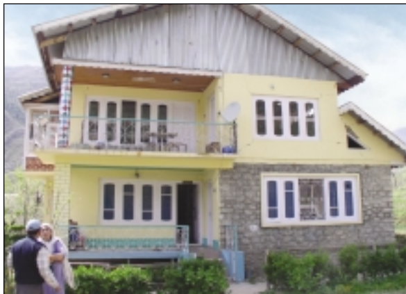
Coursed random rubble masonry without plaster
