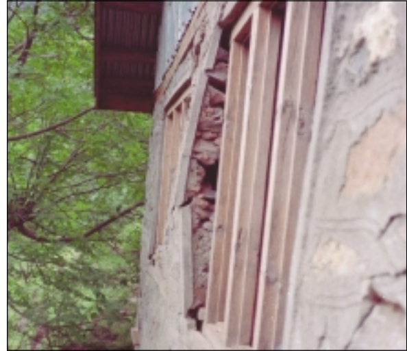
Out-of-plumb wall
