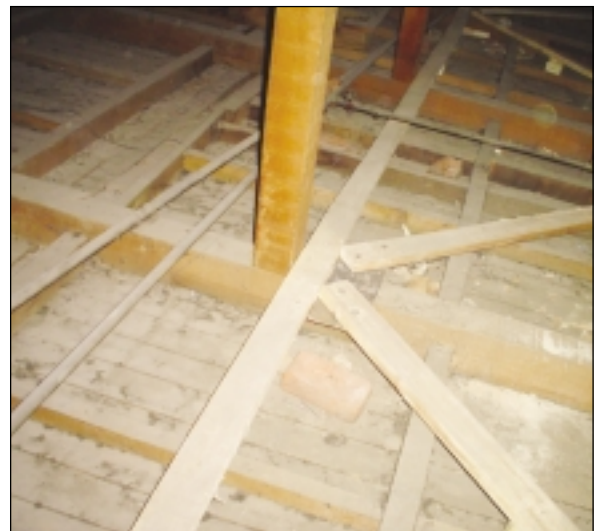
In-plane bracing & struts on attic floor
