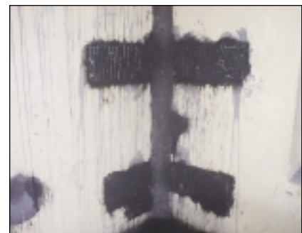
Corner crack splicing with WWM
