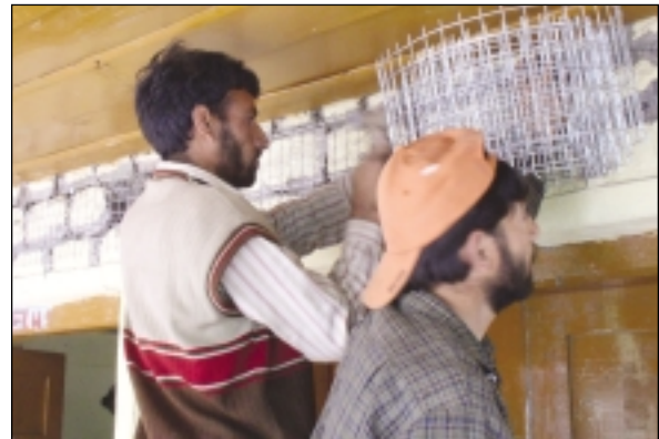
Installing WWM mesh from a roll
