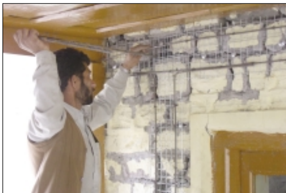
Inserting dowel for belt to belt connection at corner
