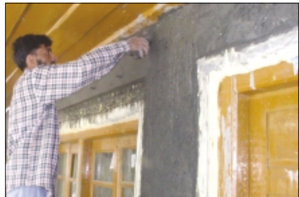
Applying cement-sand plaster
