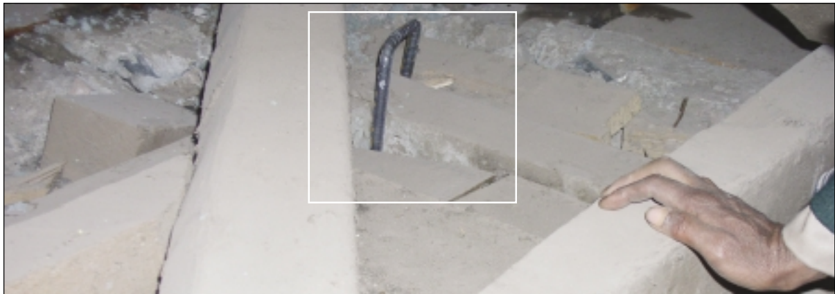
Anchoring vertical bar over wall-plate at attic deck
