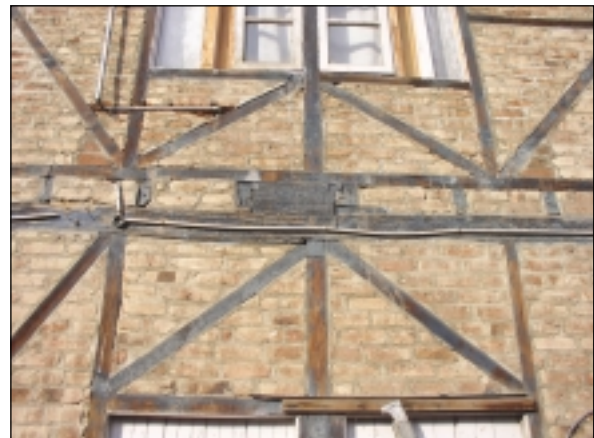
Dhajji wall with baked bricks
