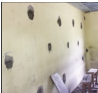
Bond elements yet to be completed in RR wall
