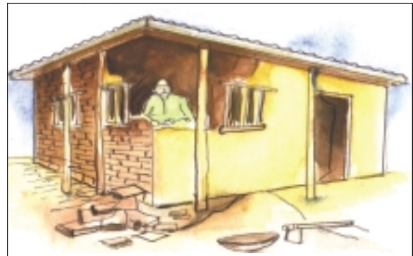
Systematically propping up slab, removing portions of damaged walls and rebuilding them
