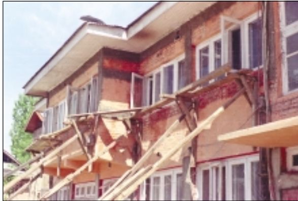
Retrofitting work in progress
