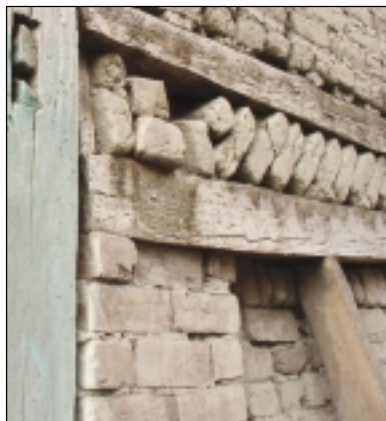
Unbaked brick wall with timber element
