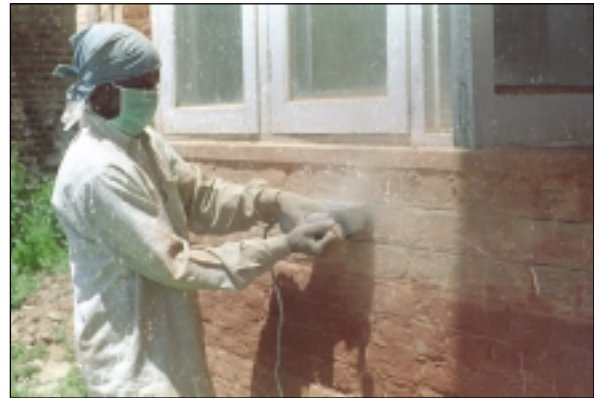
Raking mortar joints with power grinder
