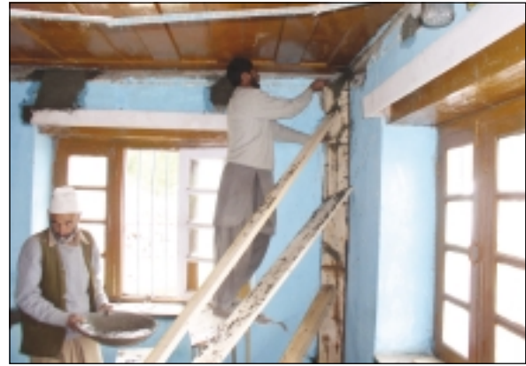
Vertical reinforcement concreting formwork
