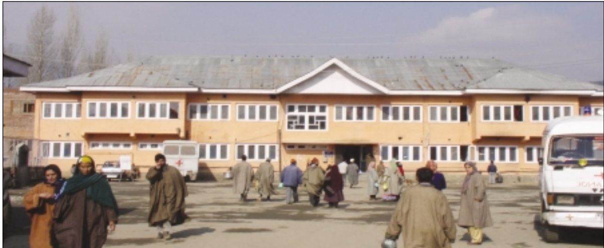
Civil hospital at Kupwada before retrofitting
