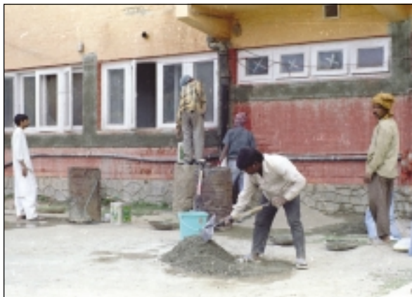
Installing WWM with bars on the walls
