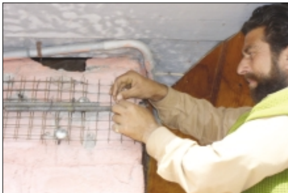
Installing 'L' shaped dowel at corner to ensure continuity
