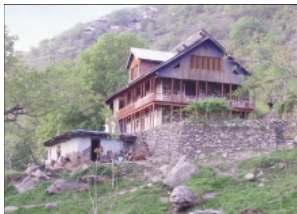
Coursed random rubble masonry without plaster
