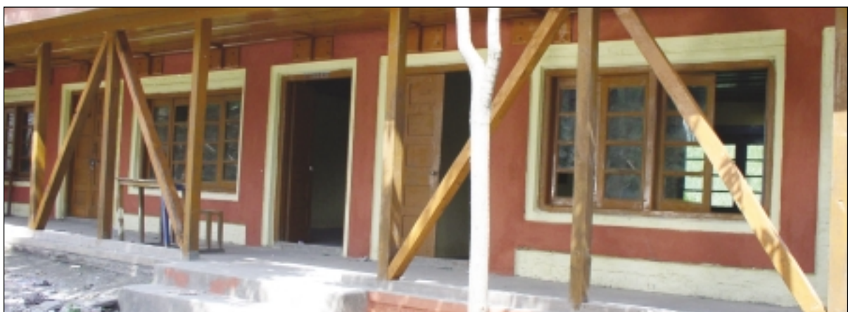
Retrofitted building with belts, roof anchoring and diagonal timber bracings
