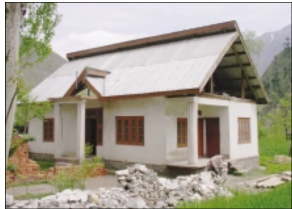
Coursed random rubble masonry with plaster
