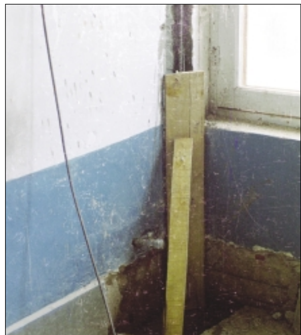
Installing vertical reinforcement at inside corners
