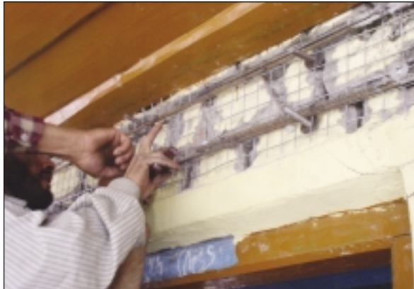
Installing bolts and brackets for roof-wall connection
