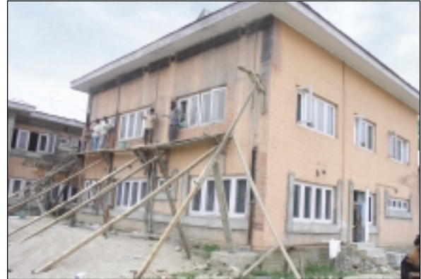
Retrofitting work in progress
