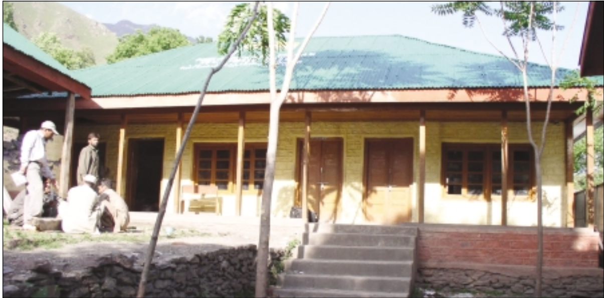
Existing 3 room school building before retrofitting
