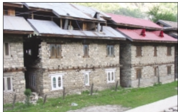
CGI sheet roofing on timber and stone masonry wall
