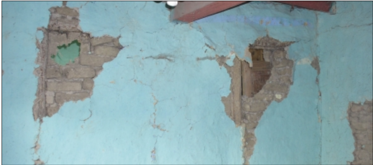
Horizontal & vertical cracking
