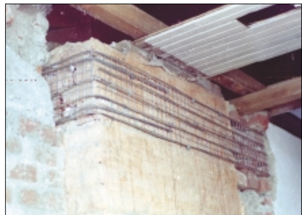
Ensuring continuity of belt reinforcement using dowels
