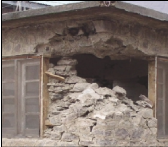
Collapsed corner
