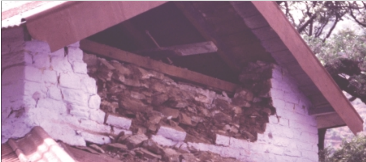
Collapsed gable wall
