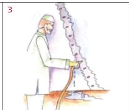
3 Injecting cement slurry
