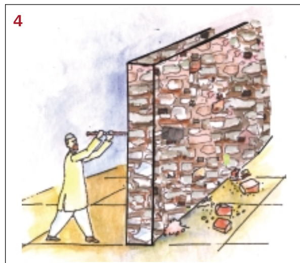
4 Pull out stone and remove loose materials behind stone
