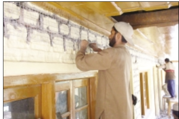
Installing belt reinforcement
