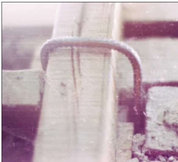
Anchoring roof wall plate corner with vertical rebar
