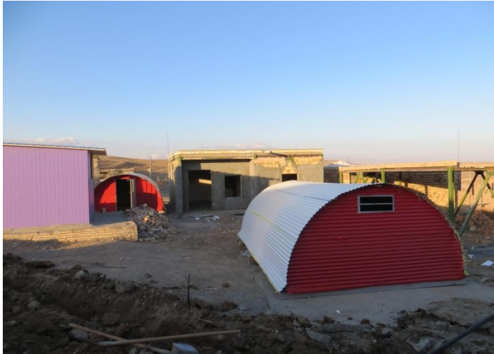
Figure 6- 24m 2 livestock shelters with curved roofing
