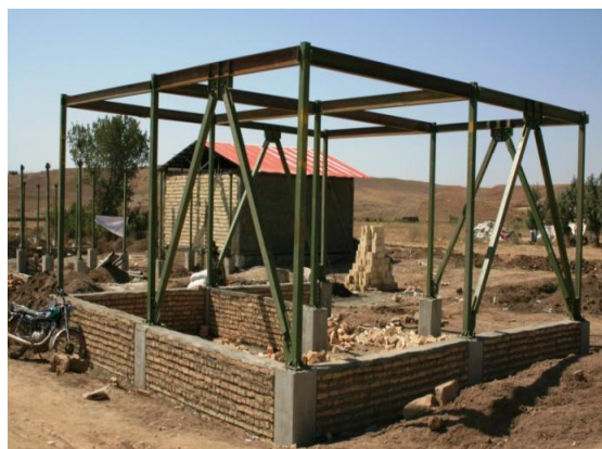
Figure 2- Steel frame with bolted connection
