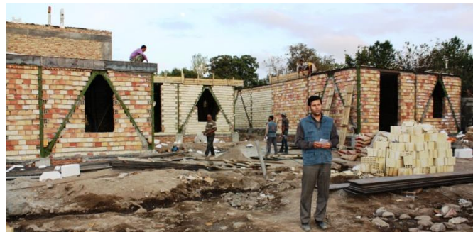
Figure 4- Typical rural permanent residential units
