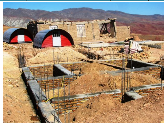
Figure 1 – Foundation close to 2 curved livestock units
