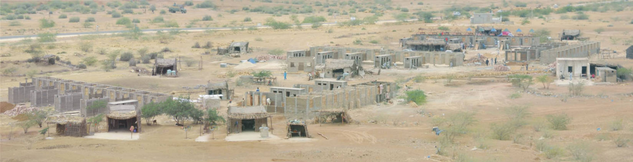
Aerial view of housing works in village Jaffar Jamari
