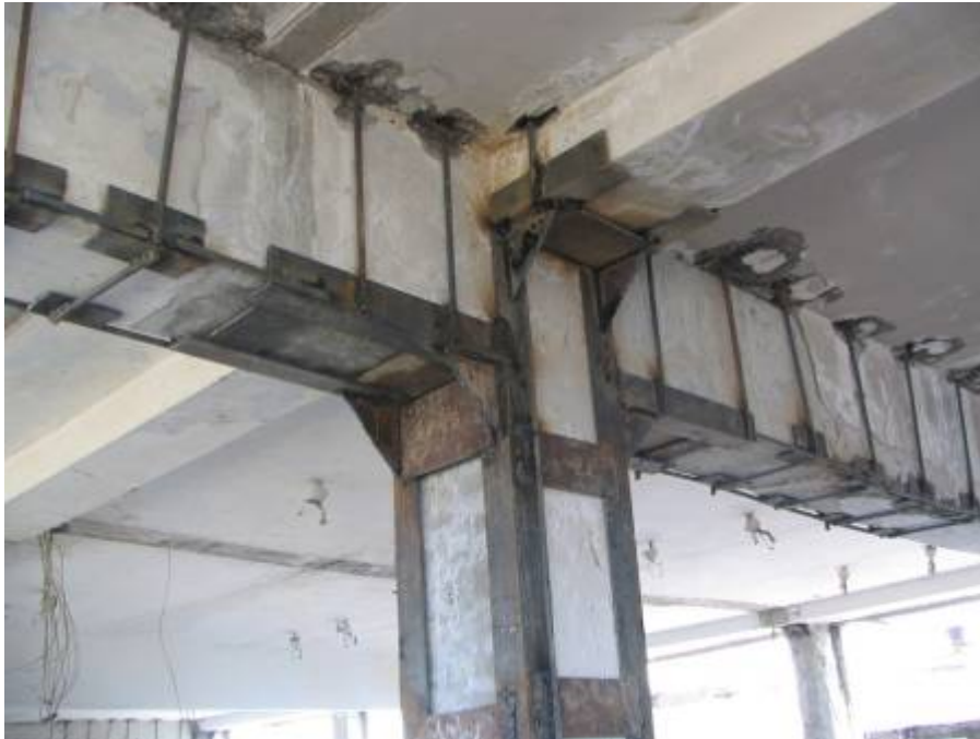
Frame-panel school N 116 in Tashkent.
