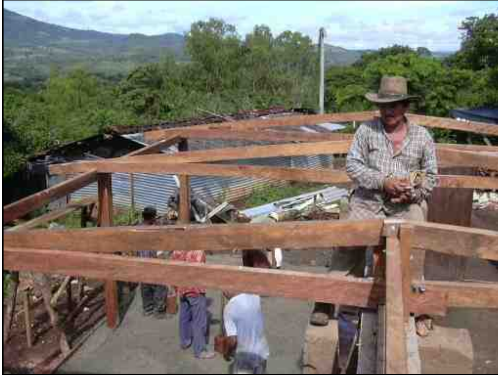
Figure 8. Roof under construction.
