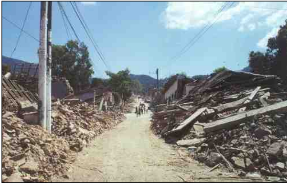
Figure 1. Destroyed adobe houses, El Salvador (López [5])
