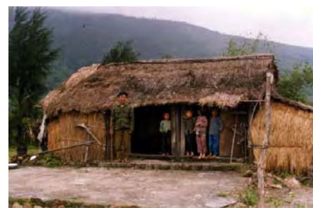
A type of house commonly found in Vietnam with little protection from flood and typhoon
