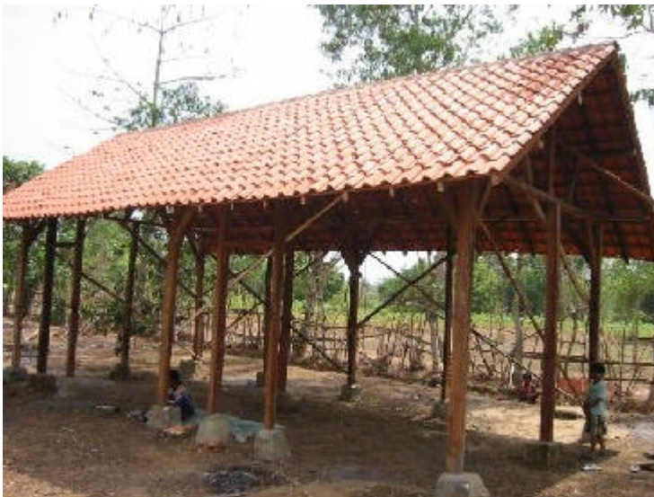
Temporary shelter with vertical structure and roof
