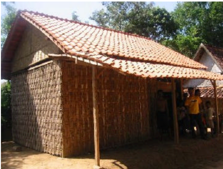
The complete temporary shelter with plaited bamboo walls
