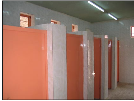
Toilets' doors after rehabilitation
