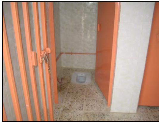
Latrines after rehabilitation.
