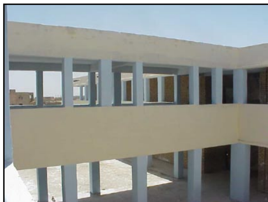
External walls after rehabilitation The work was done under UNICEF supervision
