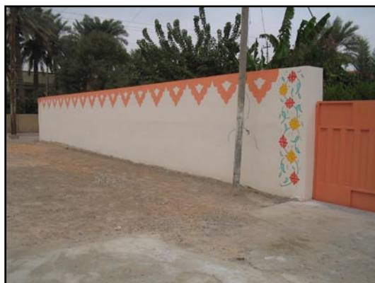
School fence after rehabilitation The work was done under UNICEF supervision
