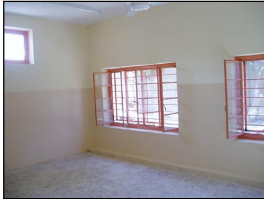
Classroom floor after rehabilitation The work was done under UNICEF supervision
