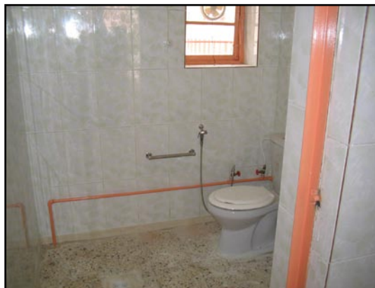
Latrines after rehabilitation
