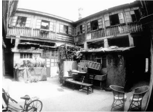
Figure 3.19 Residential Buildings at Binhai Jingqu before Upgrading
