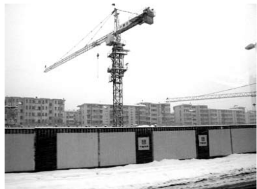
Figure 4.4. Housing Towers Financed by Developer under Construction in Binhai Jingqu Project
