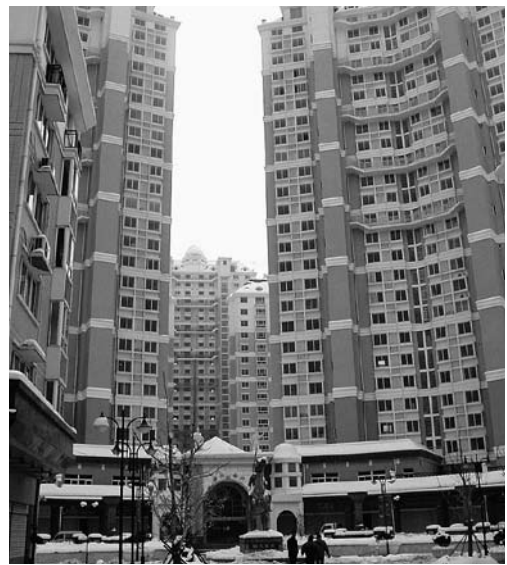
Figure 3.15 Residents' Club and High-Rise Residential Buildings in the Tongshen Redevelopment Project
