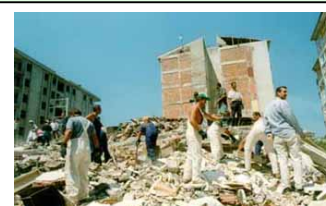
Izmit (Kocaeli) Earthquake, Turkey 1999, more than 17 000 deaths and 30% of the affected industrial park severely damaged Photo: Mikkel Oestergaard, IFRC*
