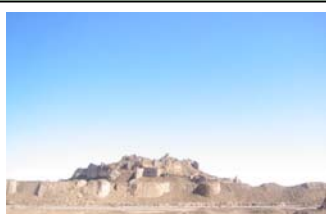
Bam Earthquake, Iran 2003, more than 25 000 deaths and the citadel (world's oldest mud brick structure) destroyed Photo: B. Rouhban, UNESCO
