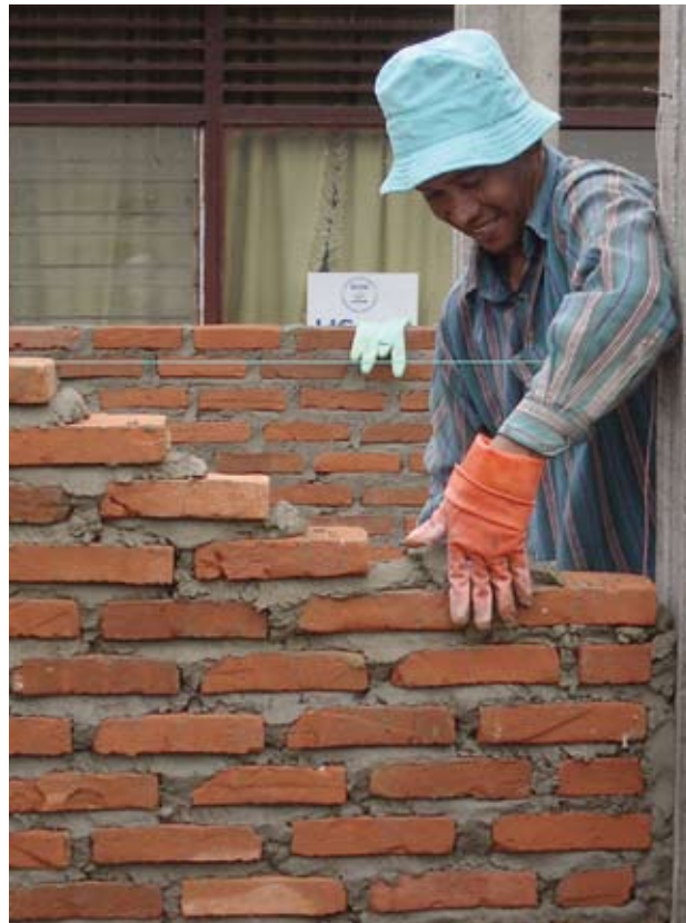
Reconstruction in Banda Aceh, using locally produced bricks
