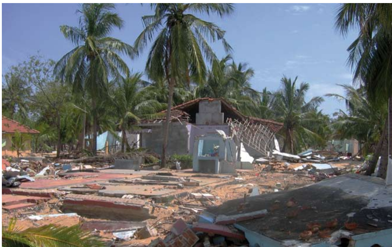
Damage from the Indian Ocean tsunami (Banda Aceh). The only thing left is the floor.
