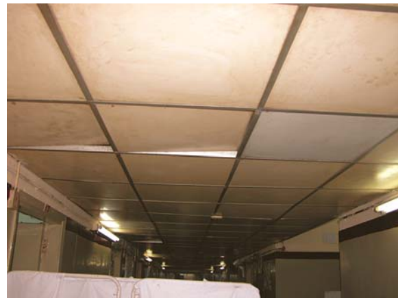
False ceiling at corridor
