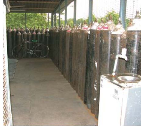
Unanchored oxygen cylinders
