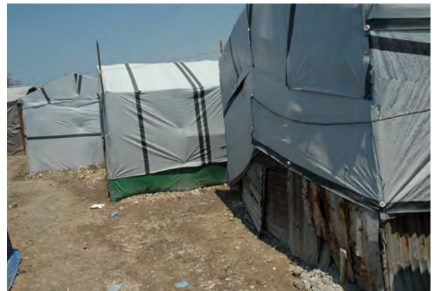
Self made shelters showing the continuous process starting with salvage materials and adding shelter plastic for roofing and weatherproofing. No technical support provided.
