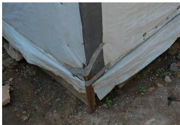
Steel peg to anchor shelter to ground, secured with hurricane straps. Pegs were relatively expensive and considered less priority by residents.
