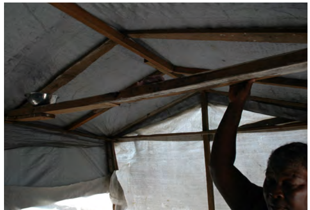
Flat roof roof upgraded to a pitched roof by carpenter support team. tie beam used to hang curtains. Higher roof also improves ventilation and thermal comfort.
