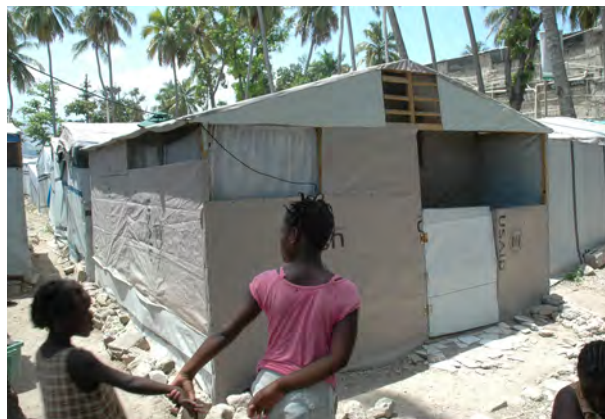
Large well framed shelter with well fixed plastic walling and windows. 'emergency shelter' which meets many of the performance criteria of t-shelter.
