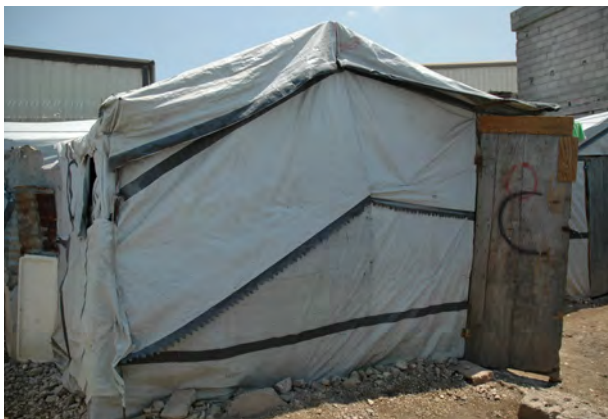
Larger shelters may require at least 2 standard plastic sheets or tarpaulins to enclose the walls and roof.
