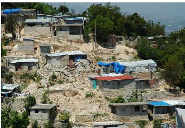
Emergency shelters constructed on the site of destroyed houses, longer term solutions may include restructuring of hazardous neighbourhoods.
