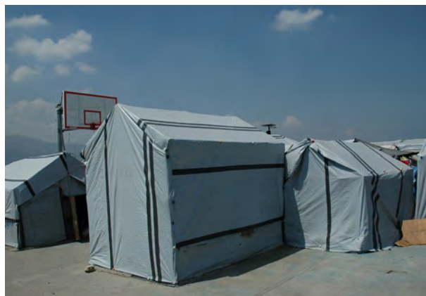
Makeshift shelters upgraded by IFRC, new plastic sheeting outside mixed material walls, to provide weather proofing as priority over ventilation and other issues.
