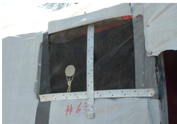
The same straps provided for hurricane reinforcement used to strengthen a window frame in a shelter. Residents used the straps in many ways.
