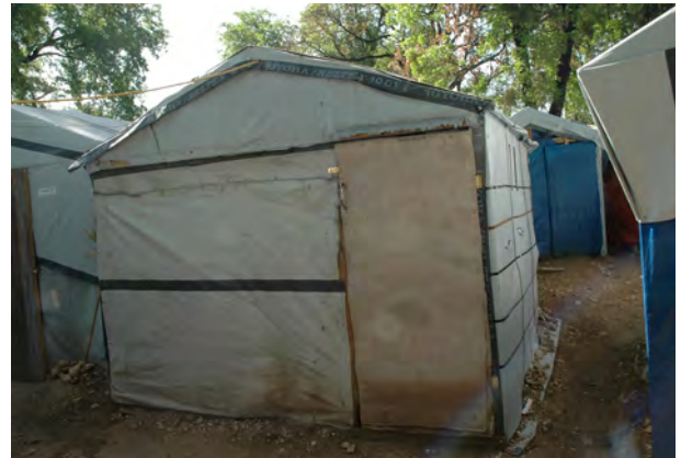
Self made shelter upgraded by CARE technical support team with material support for sheeting, framing and fixings.
