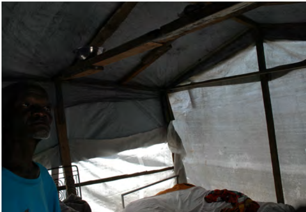
Technical support carpenter reviewing roof improvements optimising the various size timber pieces the shelter occupant had available.
