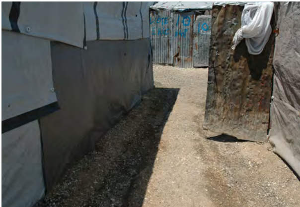
Drainage channel along the side of shelter. Low lying site at risk of slow drainage of standing water.
