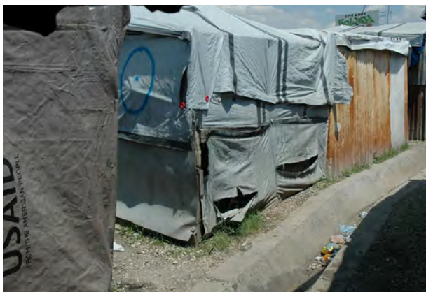
Poor quality plastic, poorly fixed and degraded. The shelter was slashed after the occupants had abandoned it.
