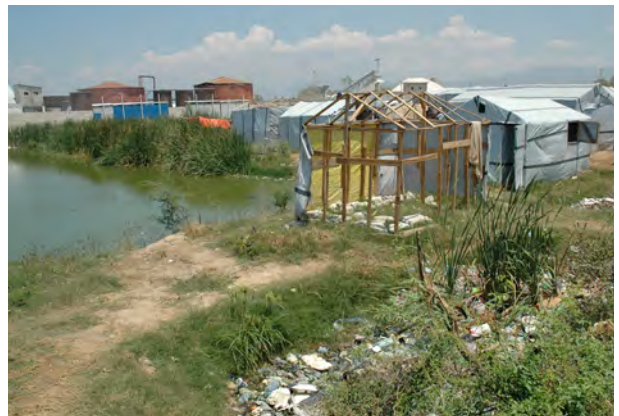
Shelters constructed on poorly drained site. Areas of the site were previously waste disposal and made ground.
