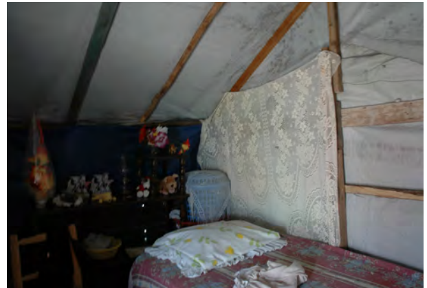
Roof and gable improved by technical support team, closer spacing of rafters.
