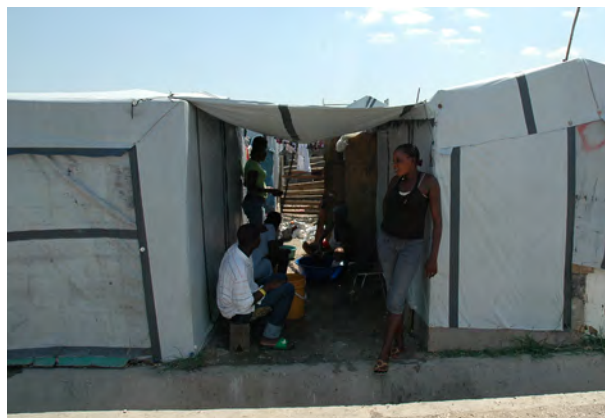
Use of plastic sheeting to cover space between shelters as additional shaded living and social space. Priorities are not only the shelter structure itself.
