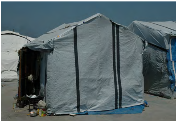
Self made shelters constructed by families with no technical support. Good local supplies of framing materials and skills. A series of distributions of plastic sheetings had taken place leading to continuous upgrading.
