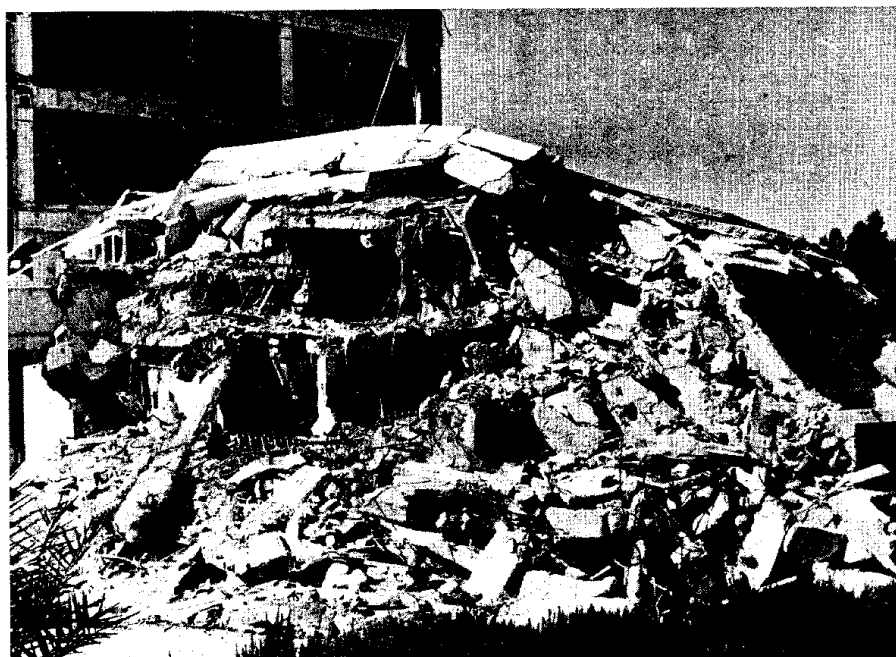
In both the southern Italian and Algerian (El Asnam), earthquakes of 1980 there was widespread damage to recently built, reinforced concrete buildings, despite the existence of aseismic building codes. This highlights the need for improved training of builders and the need for effective enforcement of building codes.
