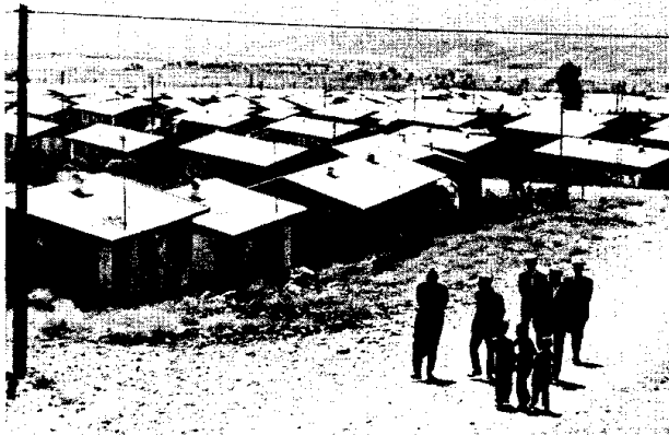
Prefabricated housing built by the Turkish Government at Lice following the earthquake of September 1975. Many families objected to the form and siting of the housing. These objections related to their lack of participation in what was provided, and the cultural and climatic unsuitability of the housing.
