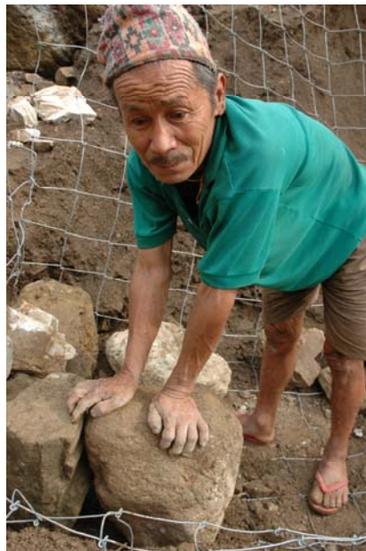
Figure 12: Loading rocks into the gabion cages, a community activity.
