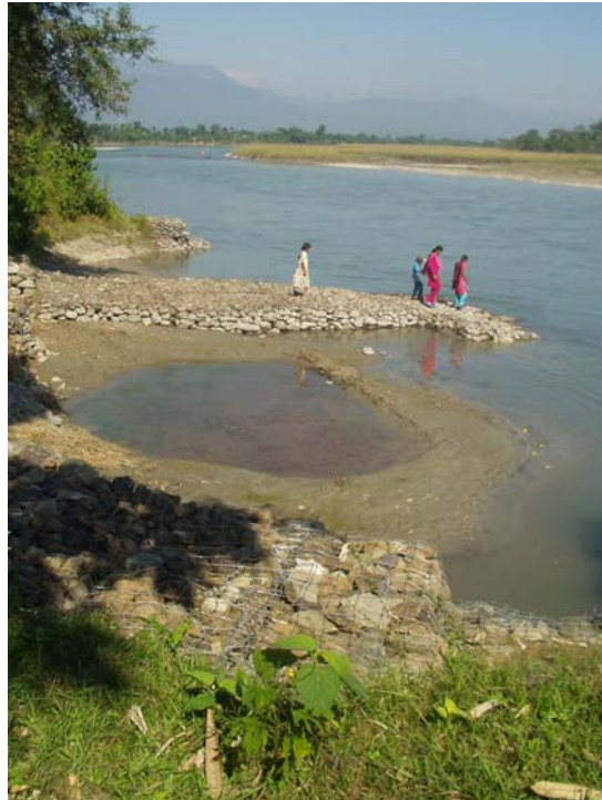
Figure 1: A small spur showing how bank erosion can be reversed by capturing sediment behind the spur. Photo: Practical Action Nepal.
