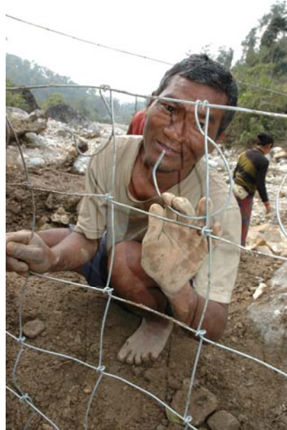
Figure 5: Making gabion cages by hand with a square mesh.
