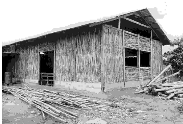
Figure 10: The Community building in Soritor during construction ©Practical Action /Rumi Velacliaga
