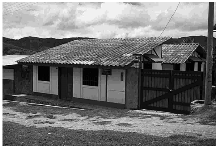
Figure 11: Improved quicha building in Jepelacio ©Practical Action /Lucky Lowe
