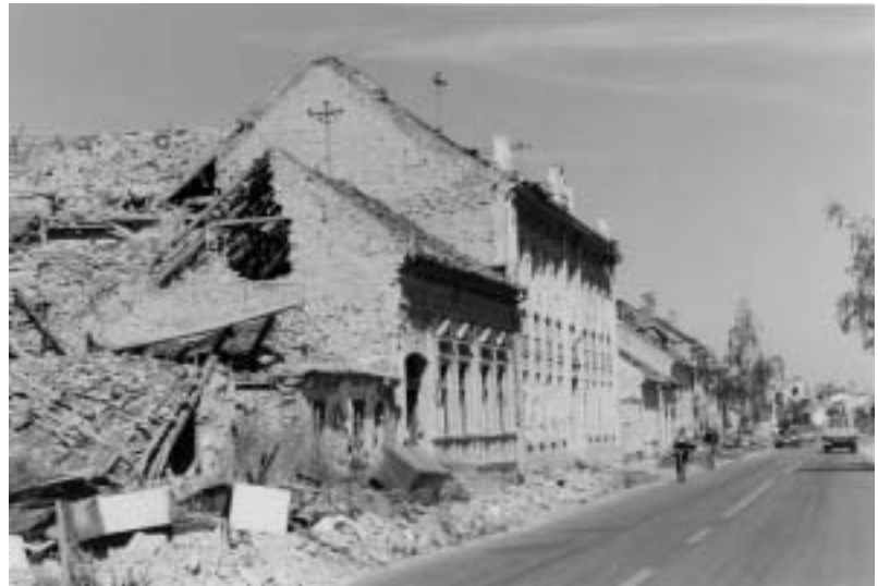
War-damaged homes, Vukovar, Croatia, September 1992
