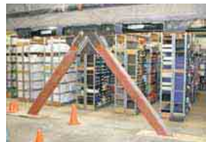
BUCKLING RESTRAINED BRACED FRAME
