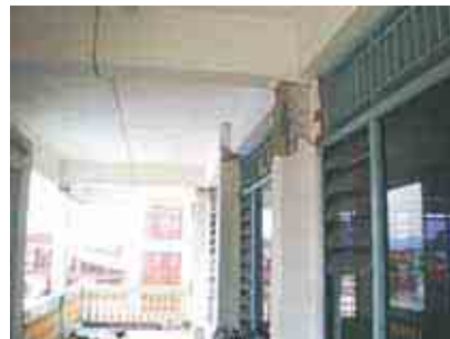
EXAMPLE OF UPPER & LOWER PARTS OF COLUMNS THAT ARE DAMAGED
