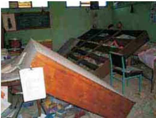
CABINETS MUST BE SAFE-GUARDED TO RESIST EARTHQUAKE SHAKING
