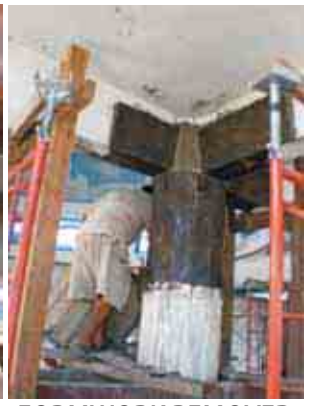
FORMWORK REMOVED AFTER CONCRETING
