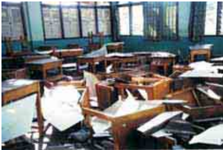
EXAMPLE OF NON-STRUCTURAL COMPONENTS DAMAGE BY EARTHQUAKE.
