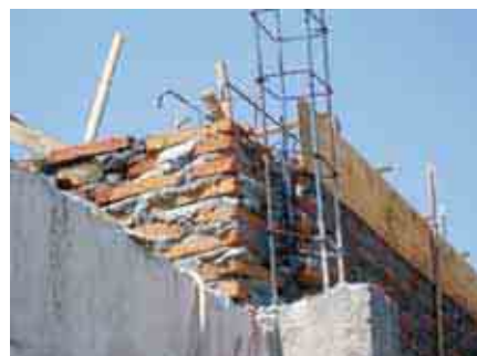
Reconstruction of School Buildings after the May 27, 2006 Yogyakarta Earthquake EXAMPLE OF POOR WORKMANSHIP
