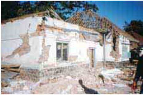
EXAMPLE OF DISLODGED ROOF TRUSSES
