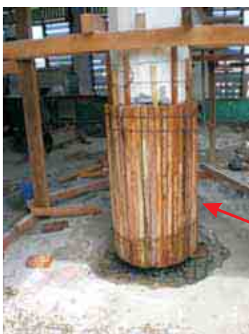
EXAMPLE OF CONCRETING UPPER & LOWER PARTS OF COLUMN
