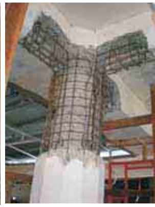
ADDITION OF STIRRUPS & ANCHORING
