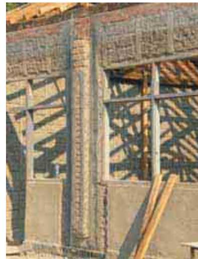
RETROFITTING SCHOOL BUILDING IN SOREANG, SOUTH OF BANDUNG USING WIRE MESH
