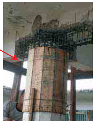
EXAMPLE OF CONCRETING UPPER & LOWER PARTS OF COLUMN
