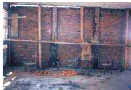
EXAMPLE OF RETROFITTING A COLLAPSED WALL
