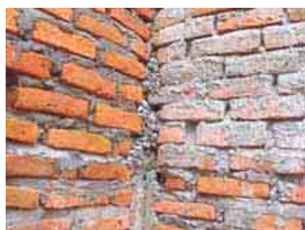
Reconstruction of Houses after the December 26, 2004 Aceh Earthquake & Tsunami EXAMPLE OF POOR QUALITY OF MATERIALS
