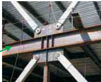
BUCKLING RESTRAINED BRACED FRAME
