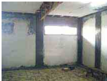
BANDAGING USING WIRE MESH
