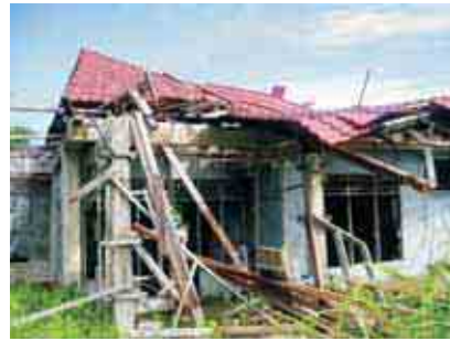
EXAMPLE OF DISLODGED ROOF TRUSSES
