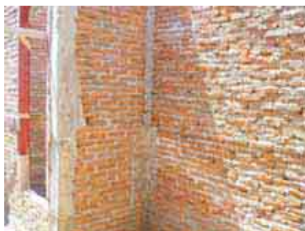
Reconstruction of Houses after the December 26, 2004 Aceh Earthquake & Tsunami EXAMPLE OF POOR QUALITY OF MATERIALS
