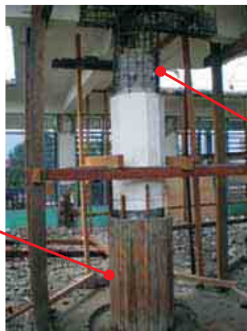
EXAMPLE OF CONCRETING UPPER & LOWER PARTS OF COLUMN
