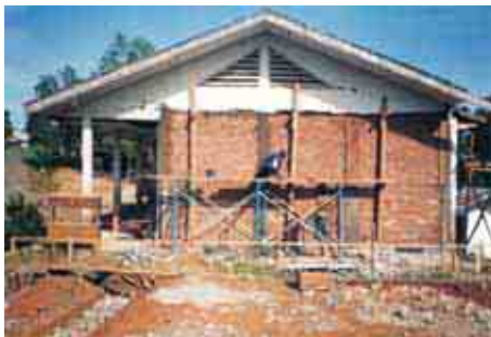
EXAMPLE OF RETROFITTING A COLLAPSED WALL
