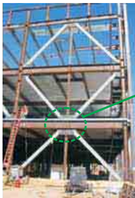
BUCKLING RESTRAINED BRACED FRAME
