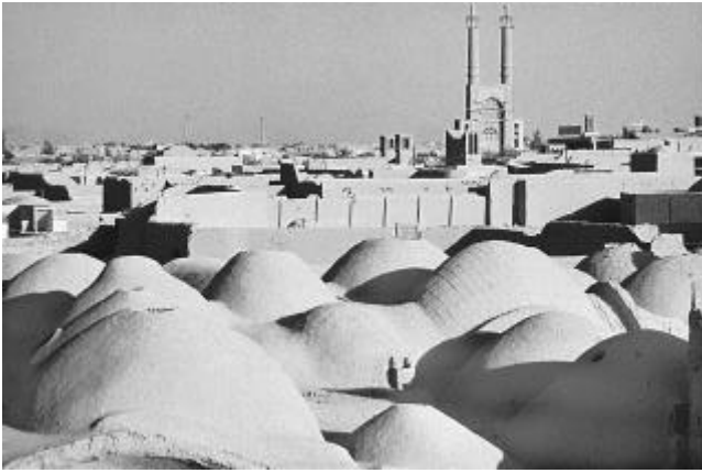
Fig. 1 Mud brick vault and dome roofscape in the traditional city of Yazd, Iran.
