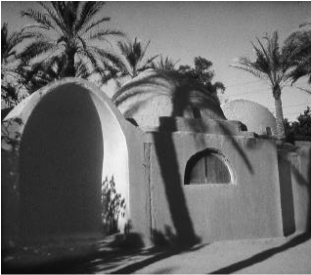
Fig. 3 The house of Hamed Said, Hassan Fathy's first building using vaults and domes in Egypt.
