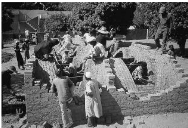
Fig. 14 Trainees practising vault building on special training structures.
