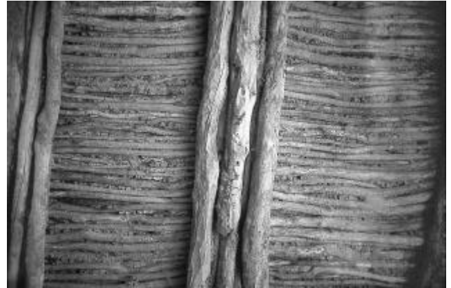
Fig. 2 Timber in a flat roof of a house in the Sahel: vast quantities of beams and branches are used.
