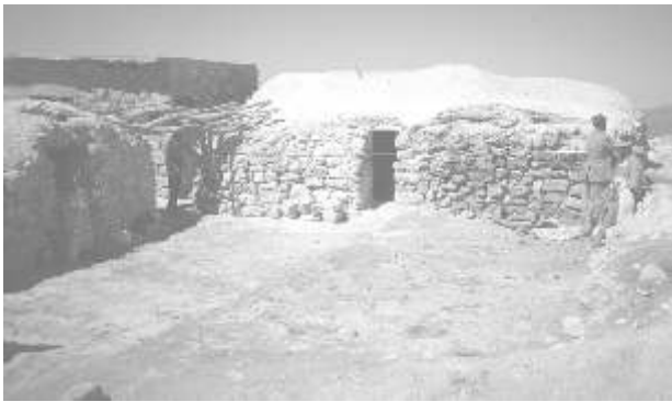
Traditional houses are built of stone with a mud roof on a wooden structure.
