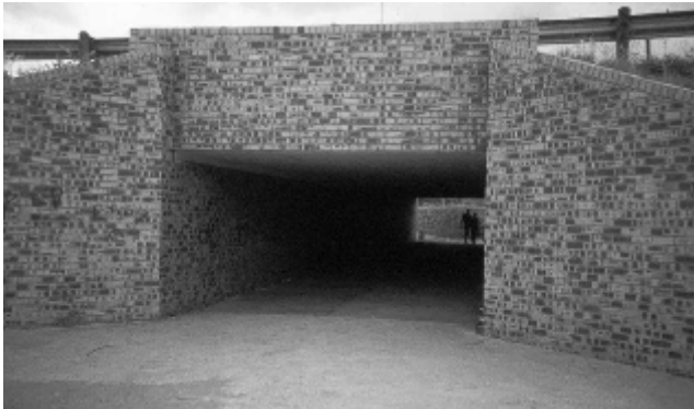
Poor design of tunnels for pedestrians may expose women to violence. Generous lightning and broad openings are necessary, if it is not possible to build a cross-over
