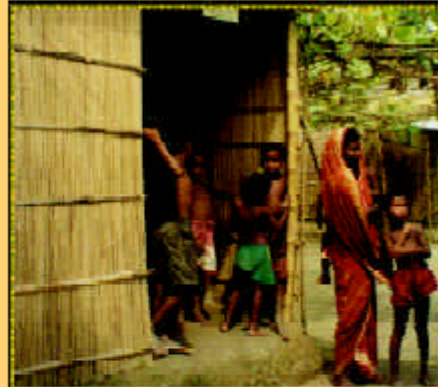
Faridpur, Bangladesh - a model house built to withstand seasonal flooding
