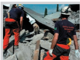
Muzaffarabad, Pakistan, A Spanish K-9 search team combs through a school when the dog signals a hit. Digging revealed 10 children dead where they had huddled for shelter, the concrete building pan caking in on them. Credit: Edward Parsons/IRIN
