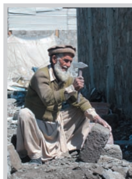
The slow, slow road to recovery. An elderly man retrieves old bricks by chipping the cement off bricks found in the rubble from the devastation in Balakot, NWFP. Credit: Chris Horwood/IRIN
