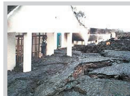
Fast-onset disasters are normally natural disasters and include cyclones, hurricanes, flooding, earthquakes, volcanoes, locust attacks and fires. In 2002 a volcano near Goma in DRC spewed lava through much of the town. Many were displaced and needed international aid. Credit: WHO
