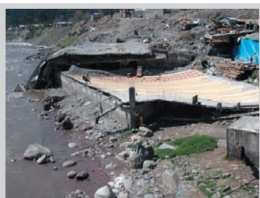
Only the courtyard remains of a huge mosque in Balakot—a town entirely destroyed by the earthquake and on live seismic faultlines. Despite the destruction prayer mats are laid out across the yard in what is an intensely religious society. Credit: Chris Horwood/IRIN
