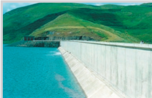
Lesotho's Mohale dam is one of the world's highest rock fill dams. $2 trillion has been spent constructing 45,000 large dams around the globe since 1900. Credit: Lesotho Highlands Development Authority
