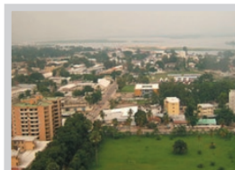
A view over Brazzaville. The government of Congo recently signed a deal with China, to improve the provision of drinking water to several Brazzaville neighbourhoods. This will require building three reservoir tanks able to hold up to 10,000 cubic meters each, which will serve 160,000 people in these neighbourhoods. Credit: Laudes Mbon/IRIN
