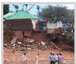
Damage caused by rain-induced floods in Hargeysa, Somaliland. Credit: IRIN
