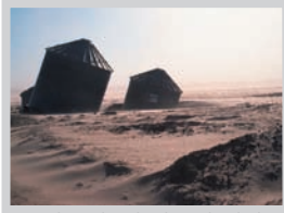
Damaged grain silos and sand covered cropland caused by a Missouri river flood, USA. Credit: Charlie Rahn/NRCS
