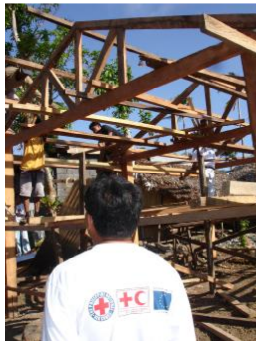
Promoting increased typhoon-resistant traditional shelter construction practices in the Philippines. International Federation
