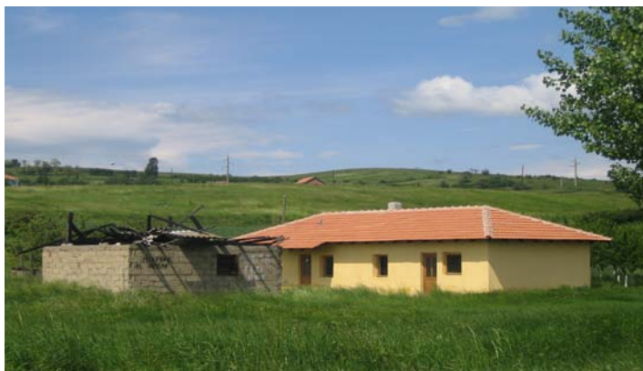
Reconstructed house next to structure destroyed in 2004 riots, Kosovo
