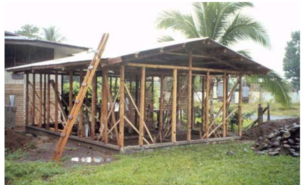
Above: PNB house under construction. Source: Gutierrez, 2000.
