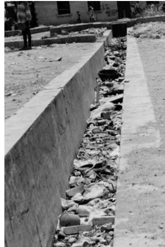
Photo: Example of Solid Waste Blocking Storm Water Drain in Accra, Ghana
