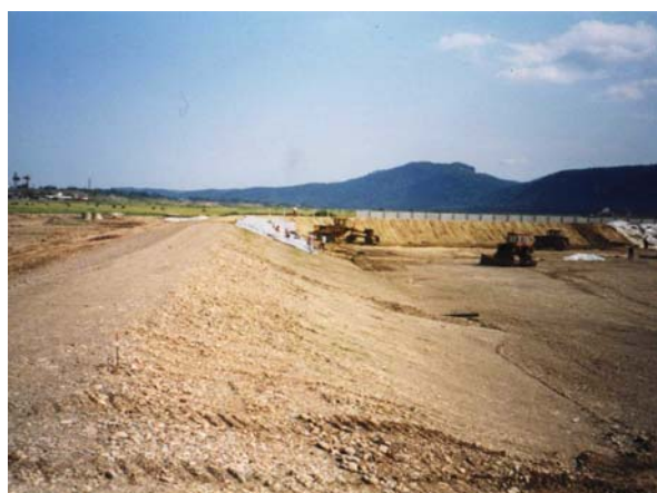
Figure: EU funded Engineered Landfill, Romania
