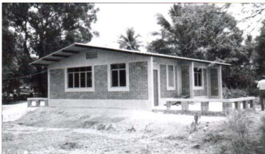
Figure 2 House built with concrete interlocking blocks
