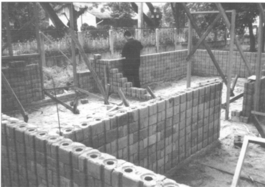
Figure 7 Typical construction site of an interlocking soil-cement block house in Thailand
