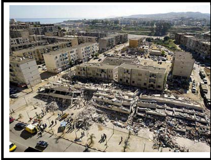
Photo 3 : Typical damage during the 2003 Boumerdes earthquake
