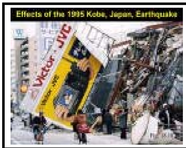
Photo 7 : Typical damage during the 1995 Kobe earthquake
