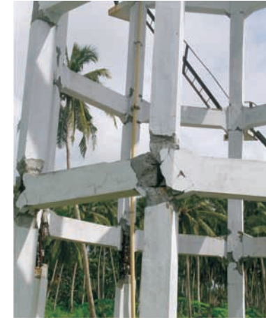
Damage to the village water tank structure
