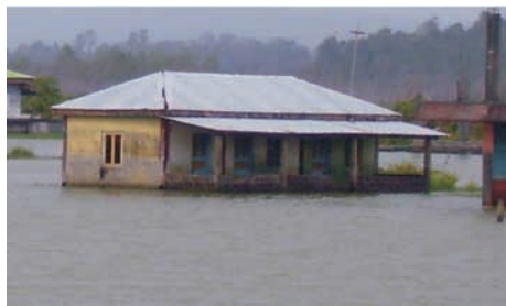
Flooding in the primary school building
