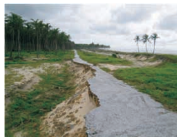
Main approach road of the village has been washed away
