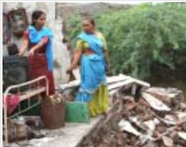
Semi-pacca house collapsed due to floodwaters damaging households as well.
