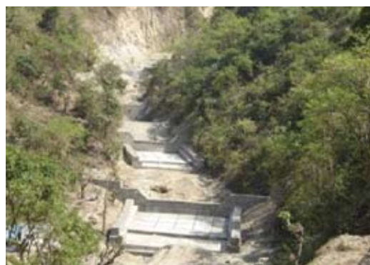
Photo 3: Check dams at Gaighat Khola at Ch 18+490 km
