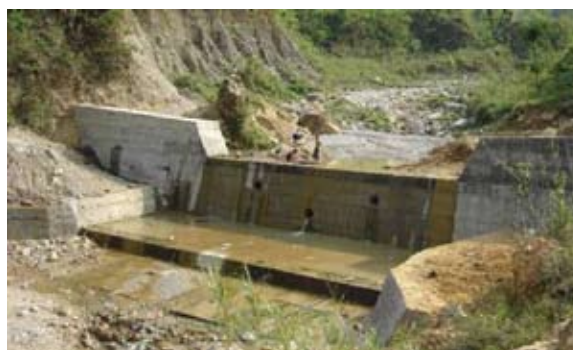
Photo 2: Sabo dam at Khahare Khola at Ch 0+220
