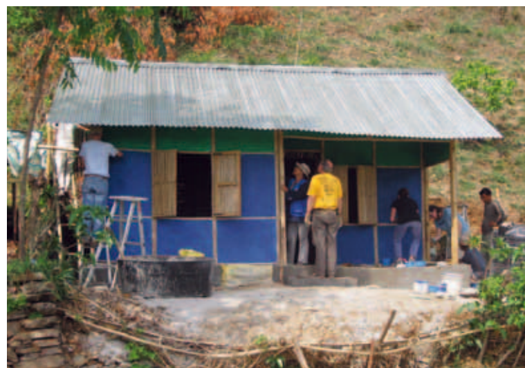
Photo3v: Habitat for Humanity dwelling under construction © UN-HABITAT
