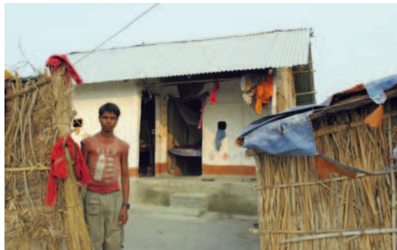
Photo10b: 235 houses were constructed by UN-HABITAT to rehabilitate landless Koshi flood victims of 2008 © UN-HABITAT
