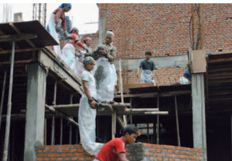
Photo3a: Owner built housing under construction in Kathmandu © UN-HABITAT
