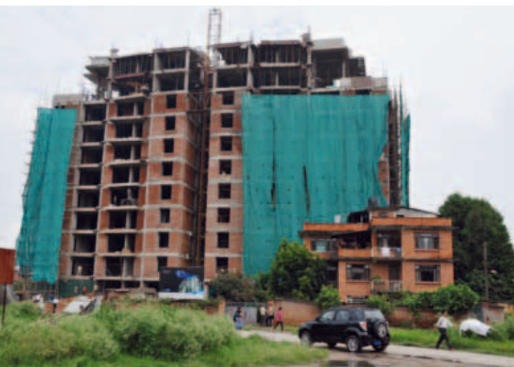
Photo3e: Apartment building under construction © UN-HABITAT
