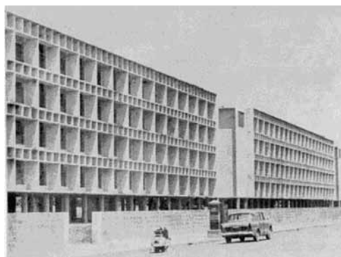
Fig.3.2: Walk-up Apartments Built in the 1960's
