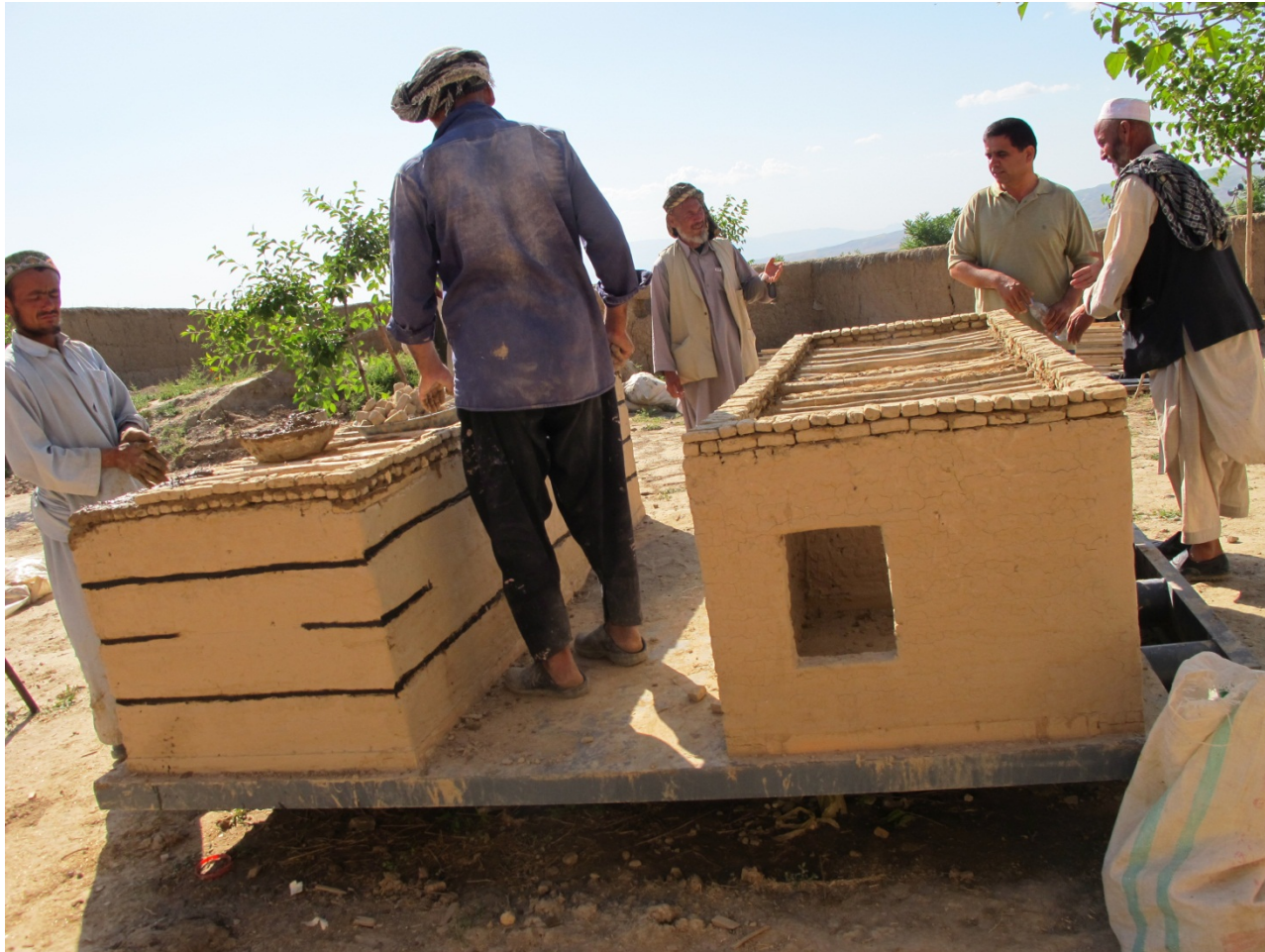
Completion of the Demonstration Units on the Shaketable
