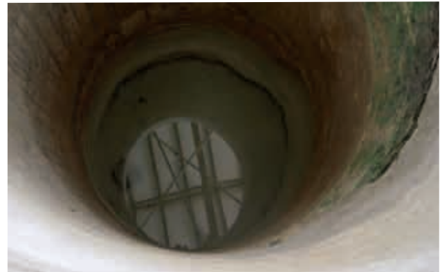
The well should be cleaned regularly!
