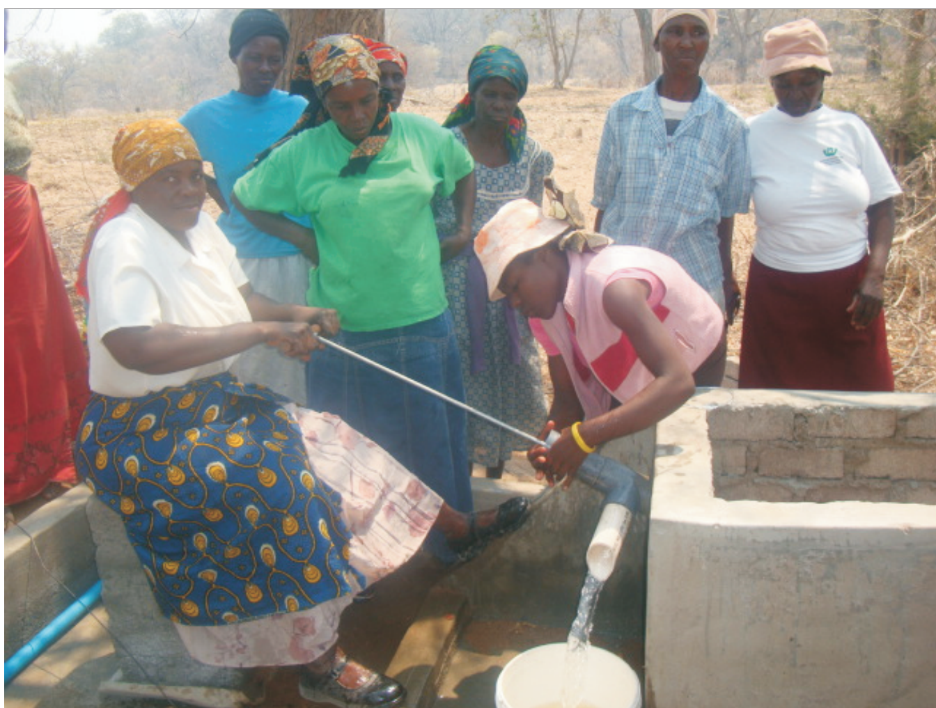
Figure 6: Women of Sivabe Garden demonstrating use of a Rowa Sand Abstraction Pump (Photo: R. Matengarufu)
