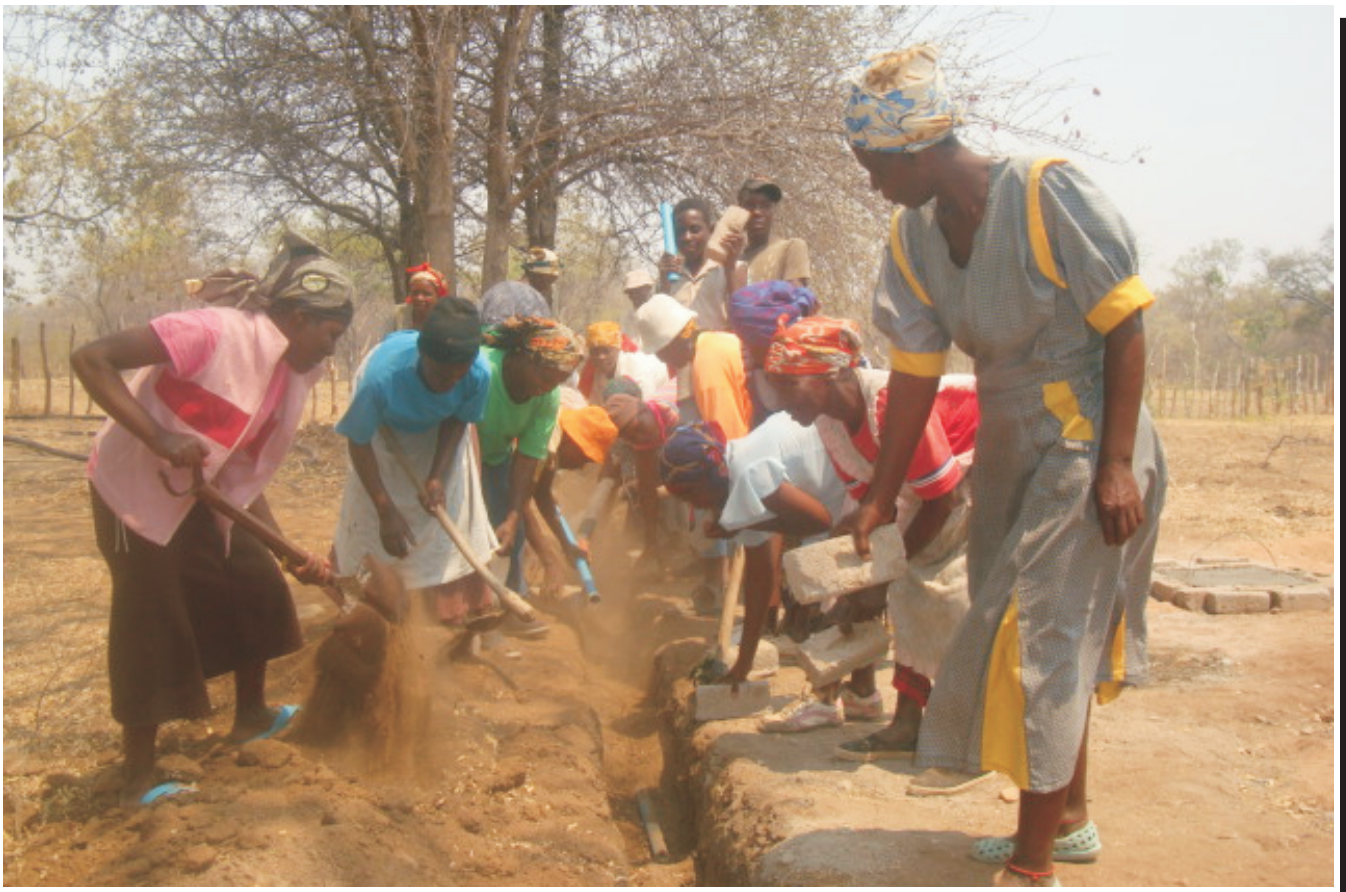
Figure 7: Sibabe Garden Sand Abstraction Pump Installation (Photo: R. Matengarufu)
